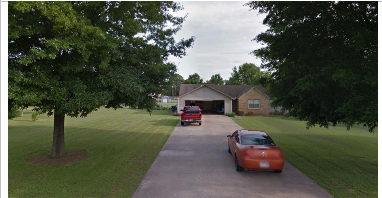
House on Jaybee Drive looking South
