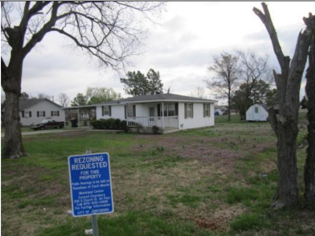
View looking northeast toward 2010 Commerce Dr. One of four subject properties.
