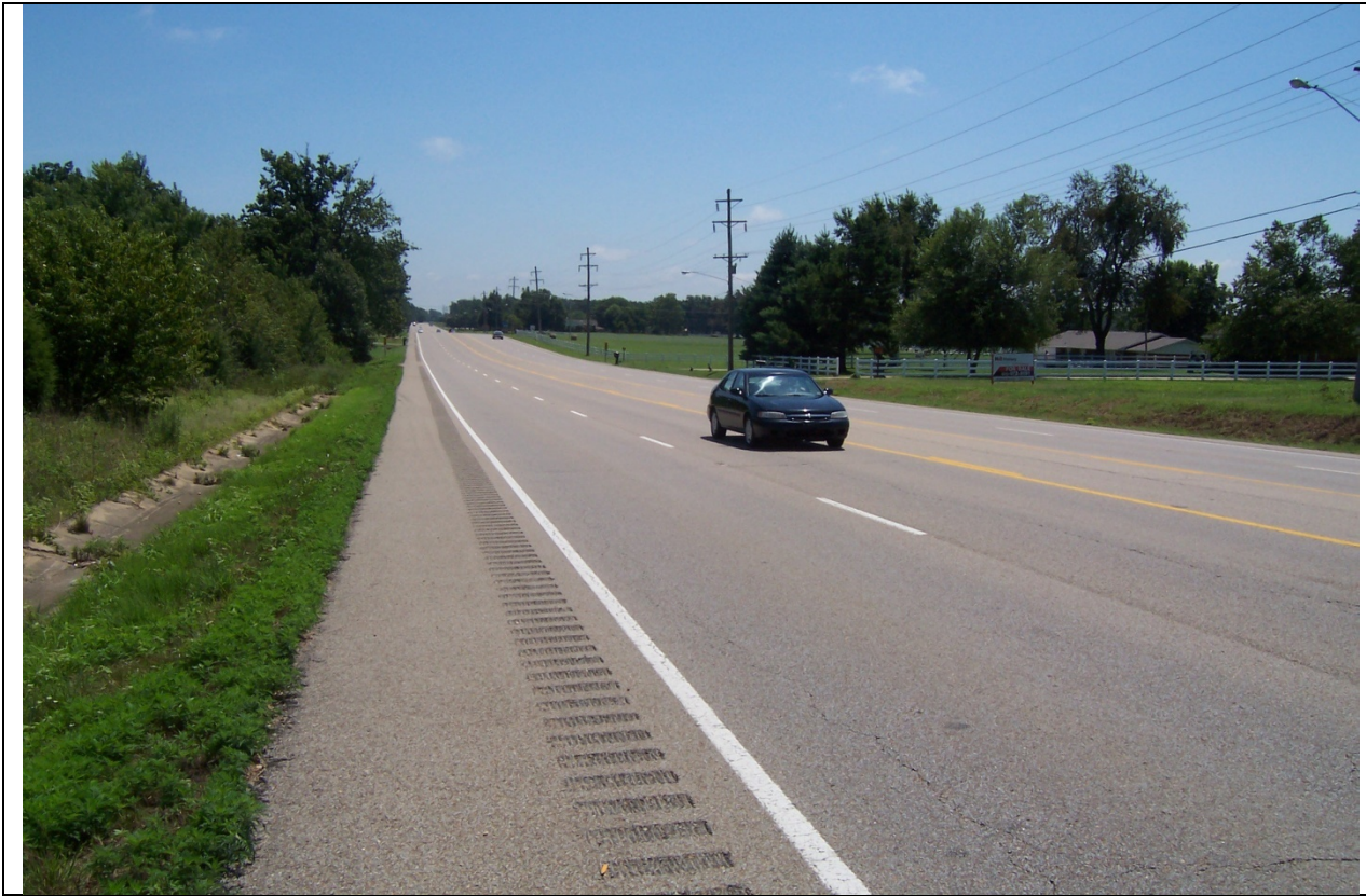
View looking East along Johnson Ave./Hwy 49.
