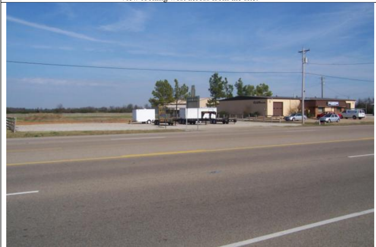
View looking northeast at the subject site.
