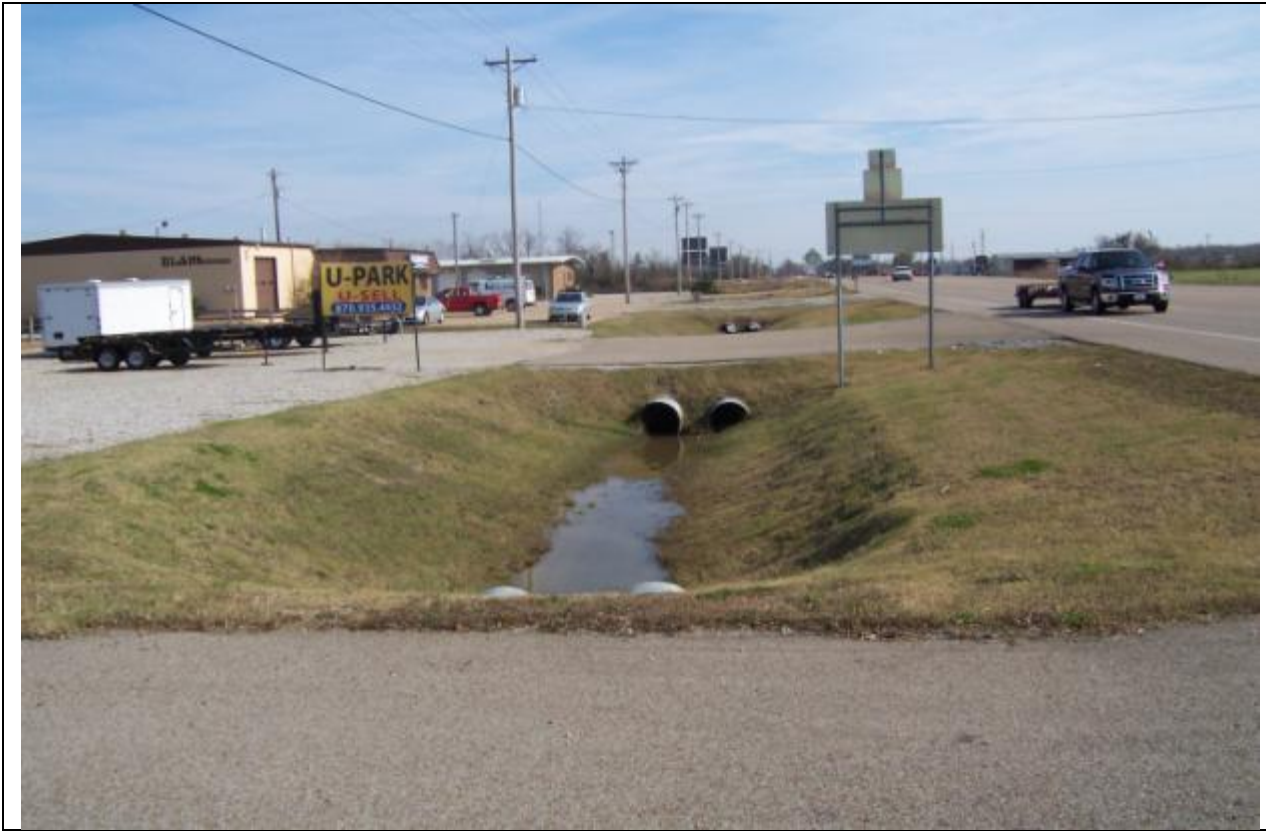
View looking east from the site.
