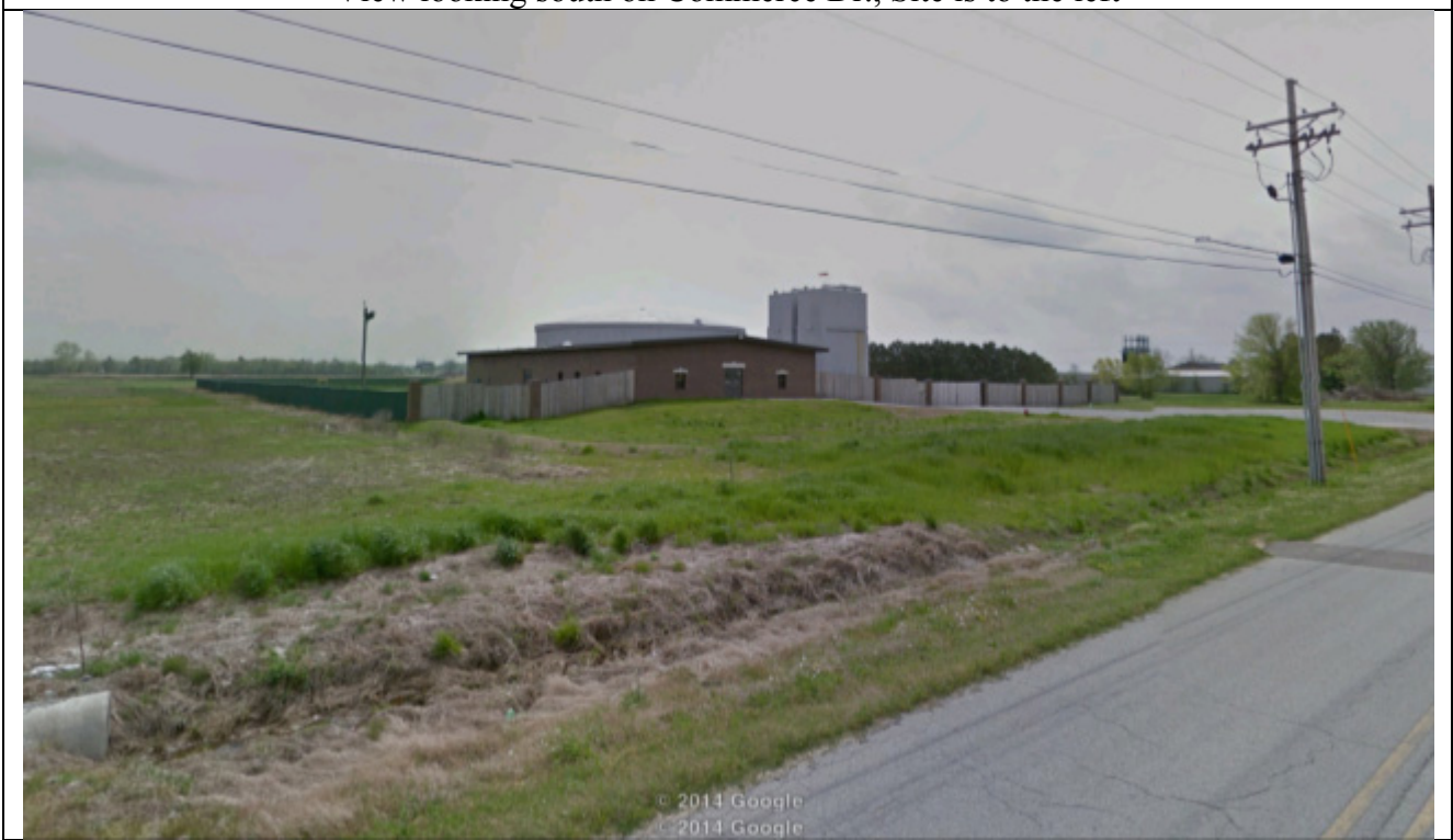
View looking southeast at City Water & Light Plant
