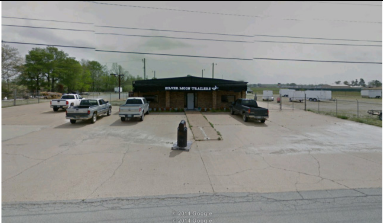
View looking east toward subject property
