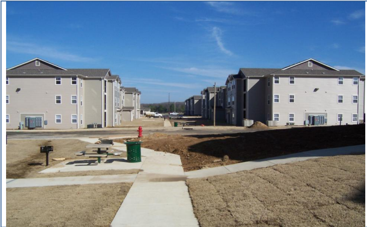
View looking East within the Willow Creek Apartments complex.
