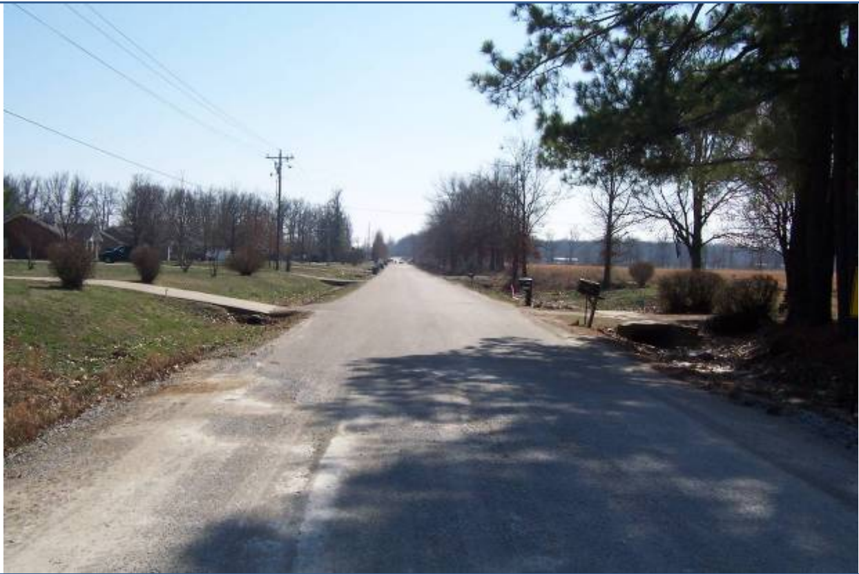
View looking South along Clinton School Rd.(South of Subject Property)
