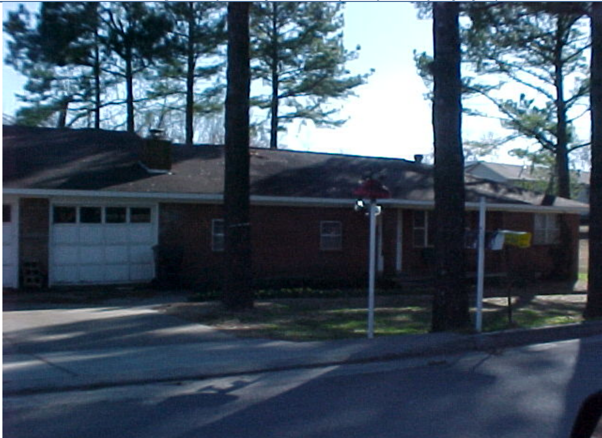
View Looking South at Subject Non-Conforming Structure/Home
