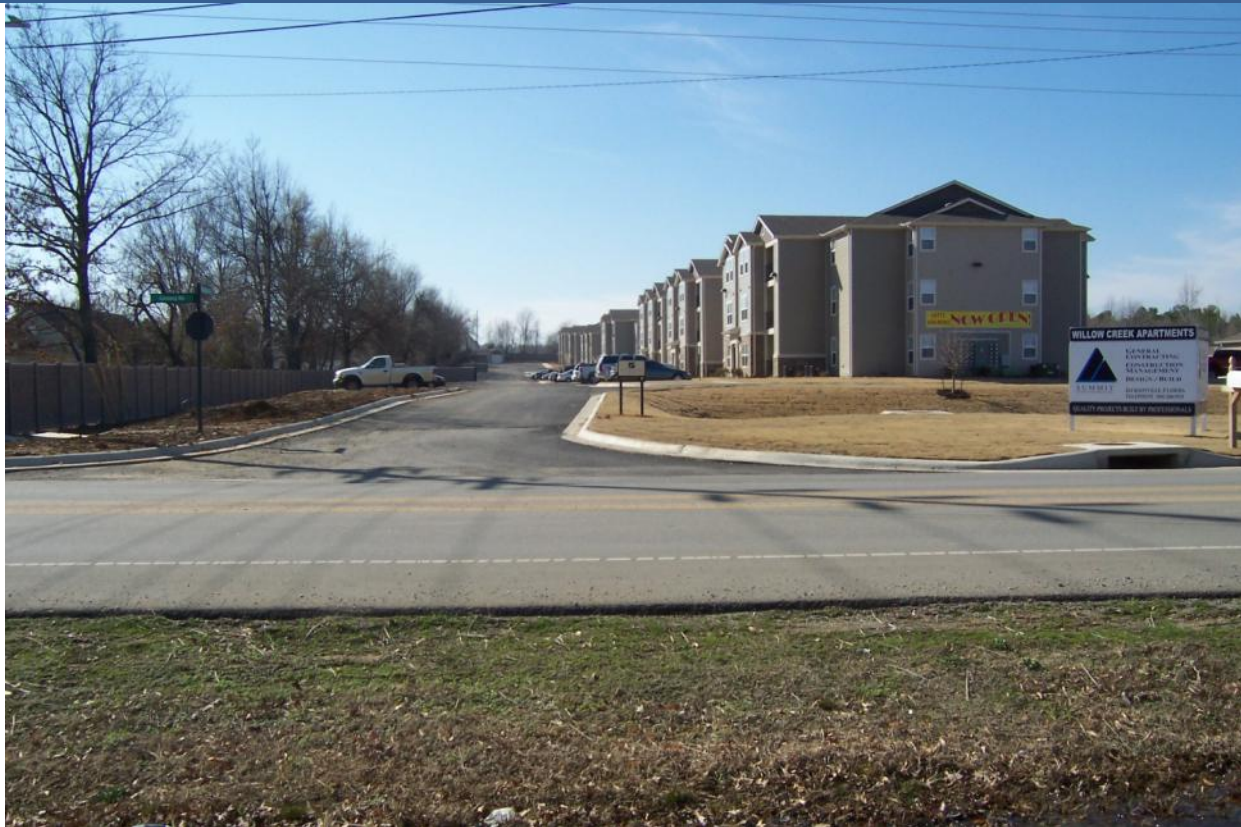
View looking West of apartment entrance (south).
