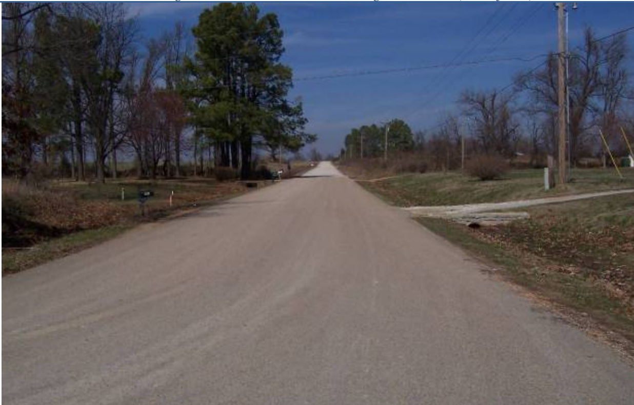
View looking North along Clinton School Rd. (CR701)
