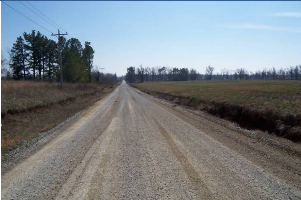
View looking South along unimproved CR701 (Site to left)
