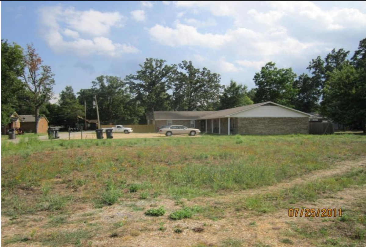
View looking South of abutting apartment complex.
