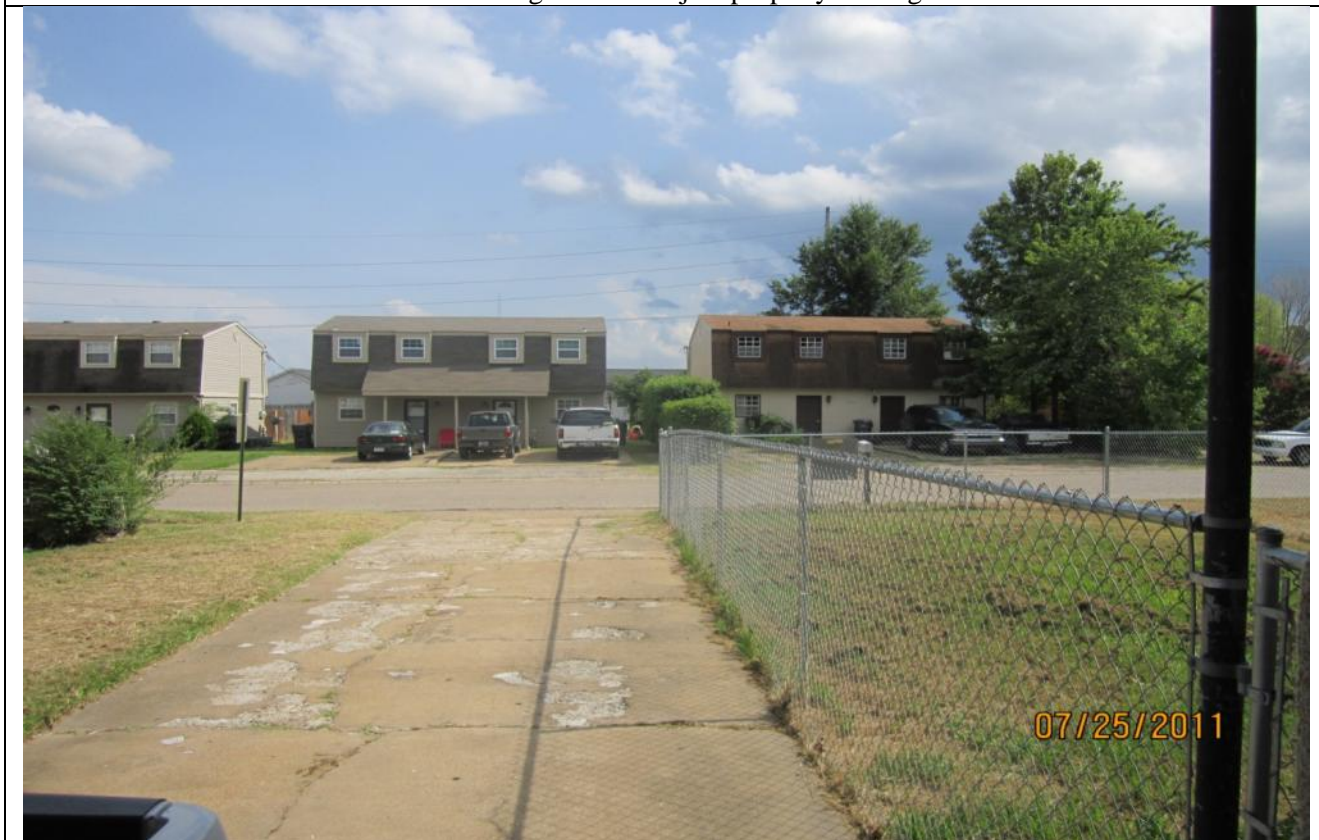
View looking South from site of multi-family dwellings.
