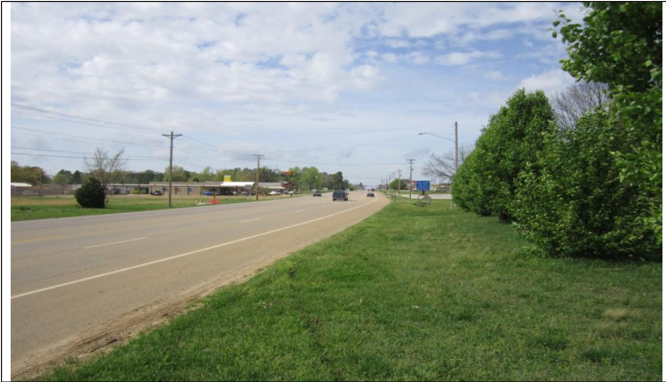
View looking easterly along Highway 49N
