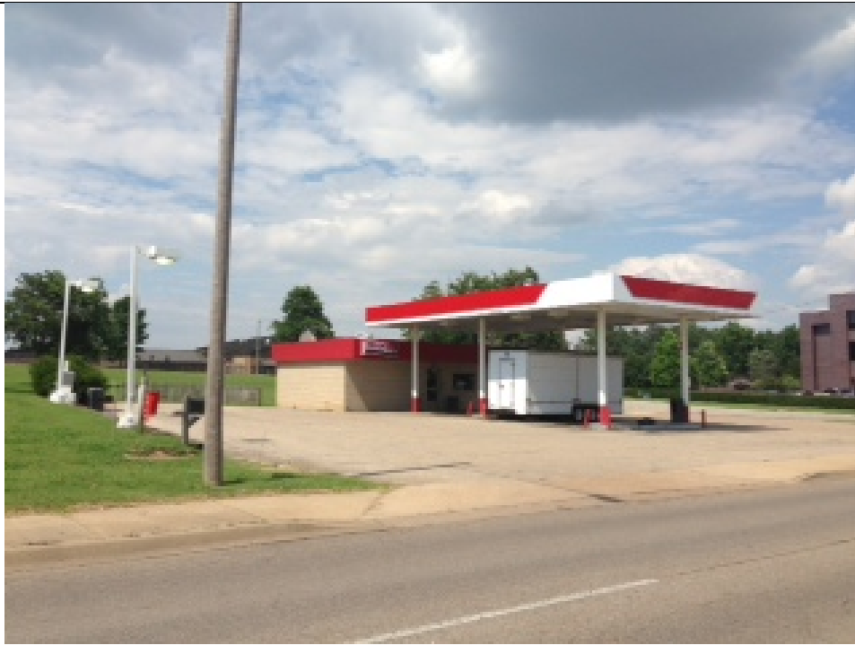
View looking Northeast towards site
