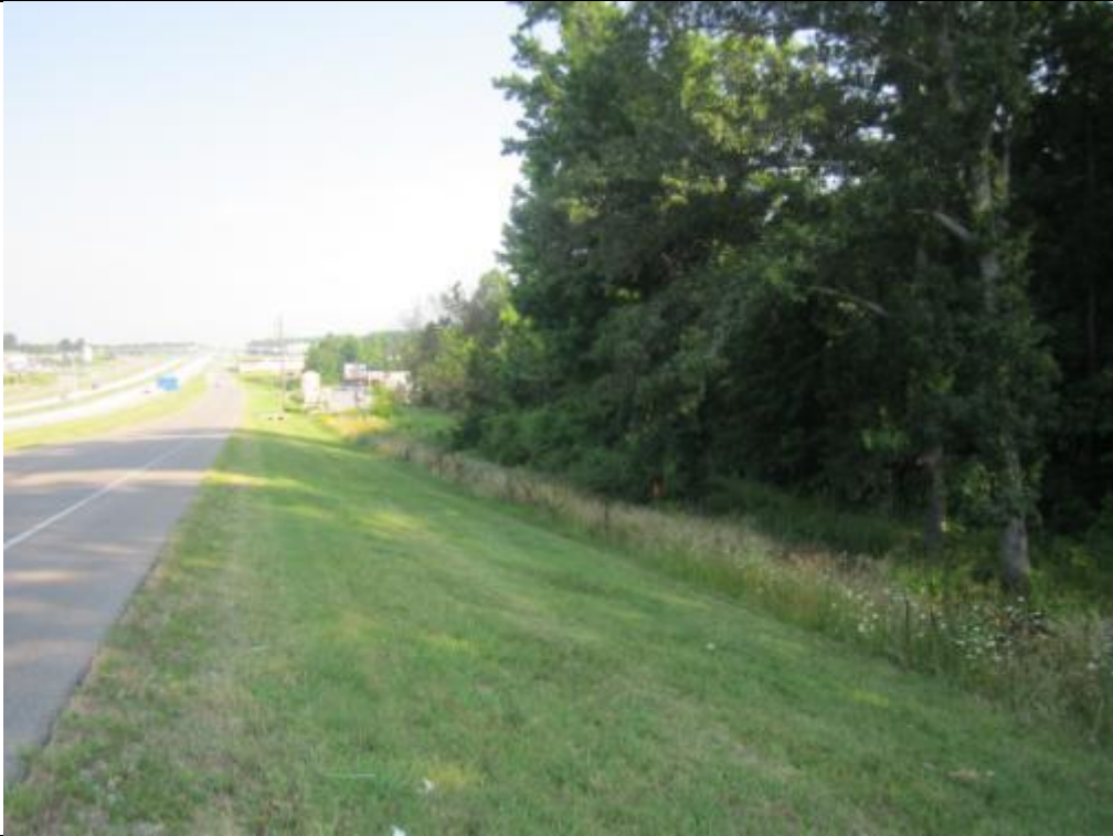
Southeast corner of site viewing northwest along Alexander Drive.
