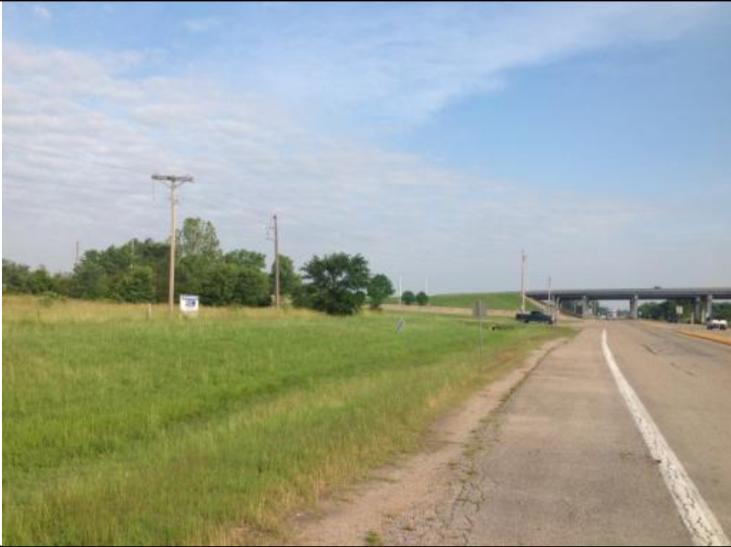
View looking North towards I-63 / I-463 Interchange
