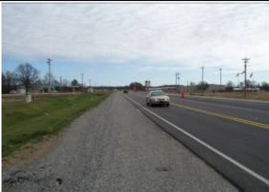
View Looking East along Hwy 49
