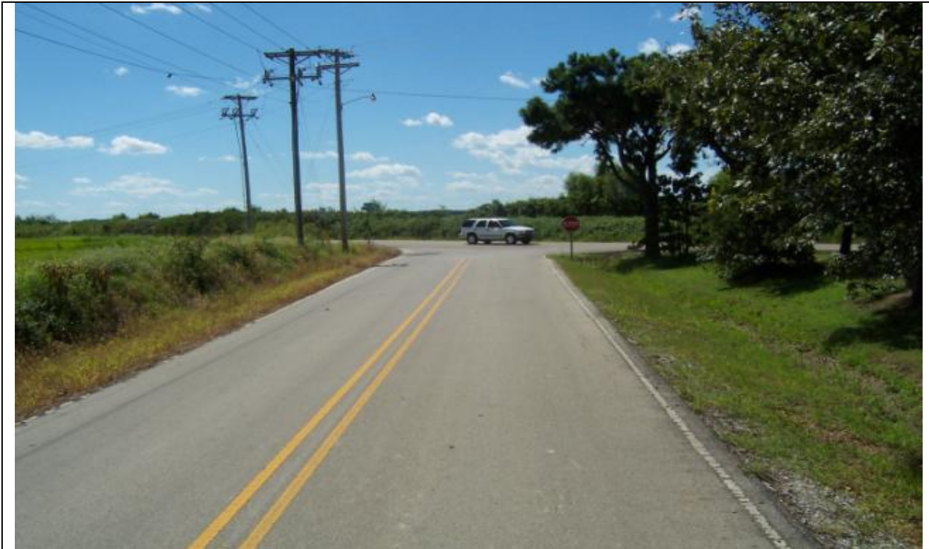
View looking west along Pacific Rd.
