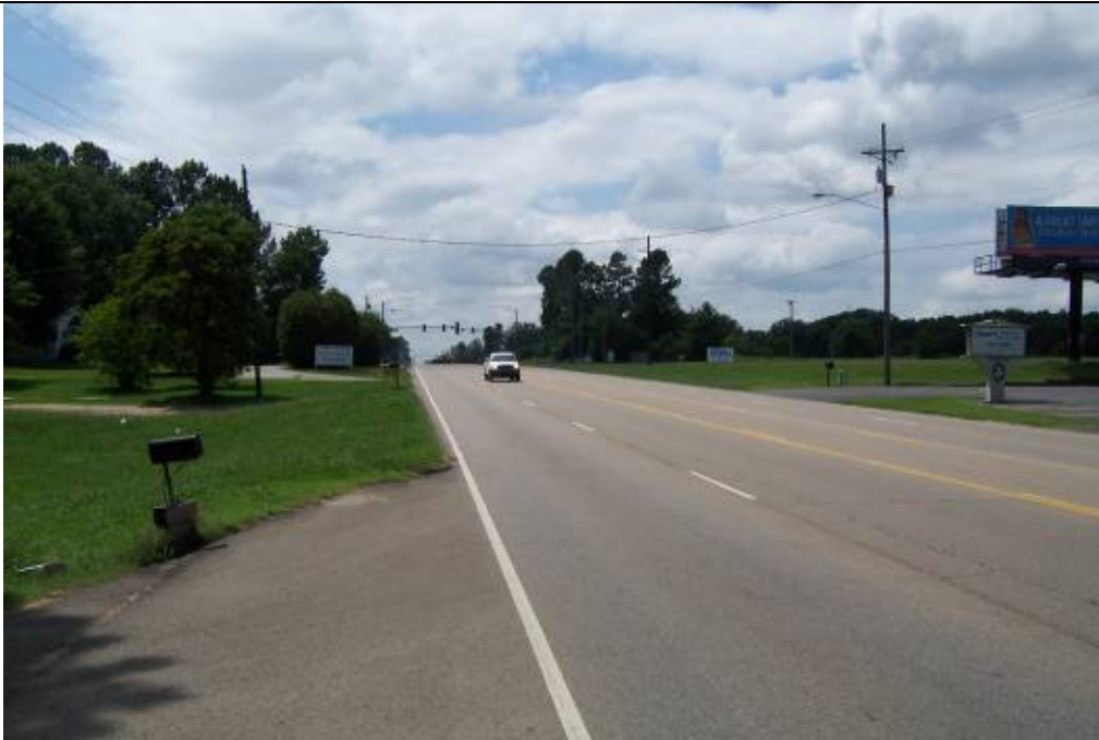
View looking southwest from site.
