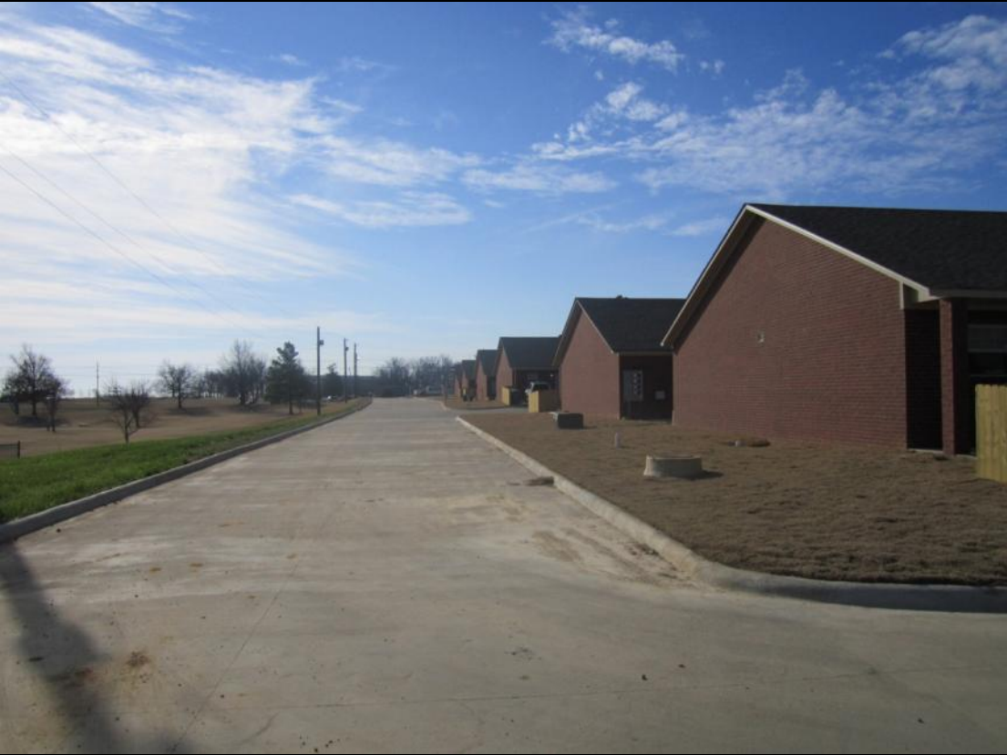
View looking South from rear of Higgins property Lot 2.
