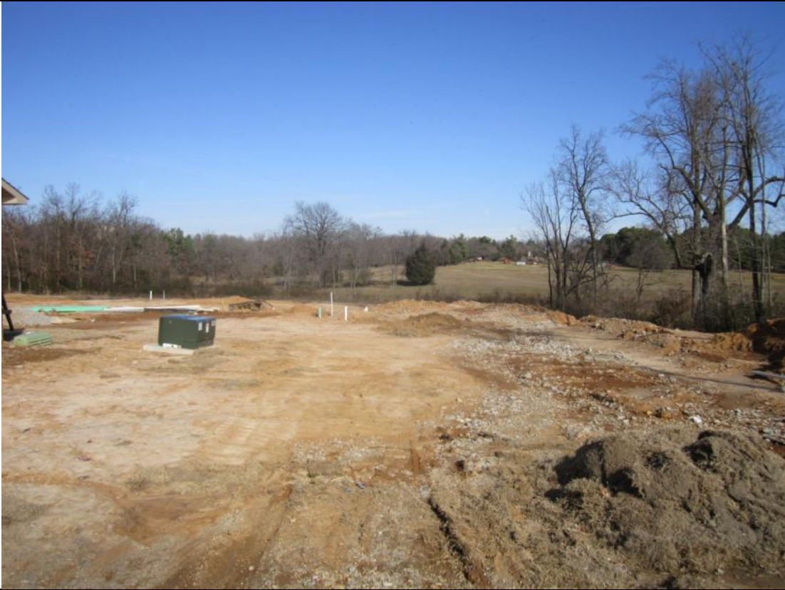
View looking North new apartments of vacant lots.
