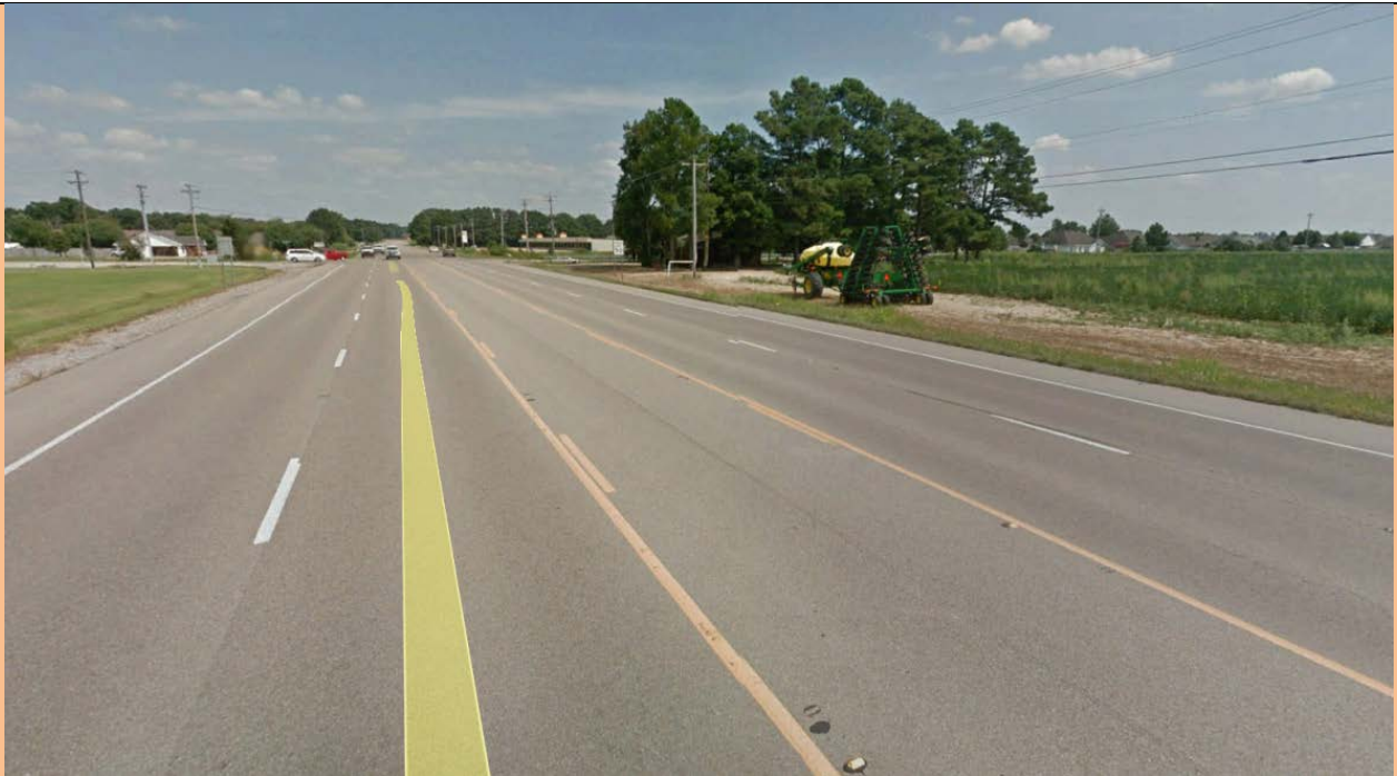
View looking East
