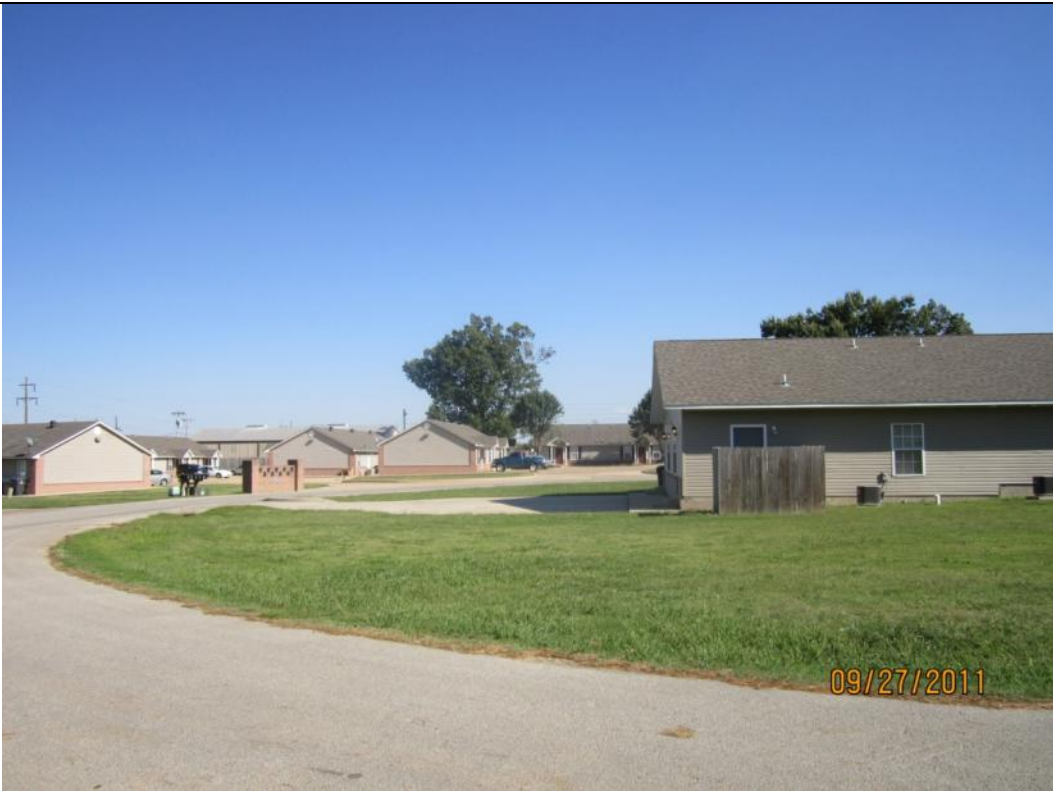
View looking East of additional apartments.
