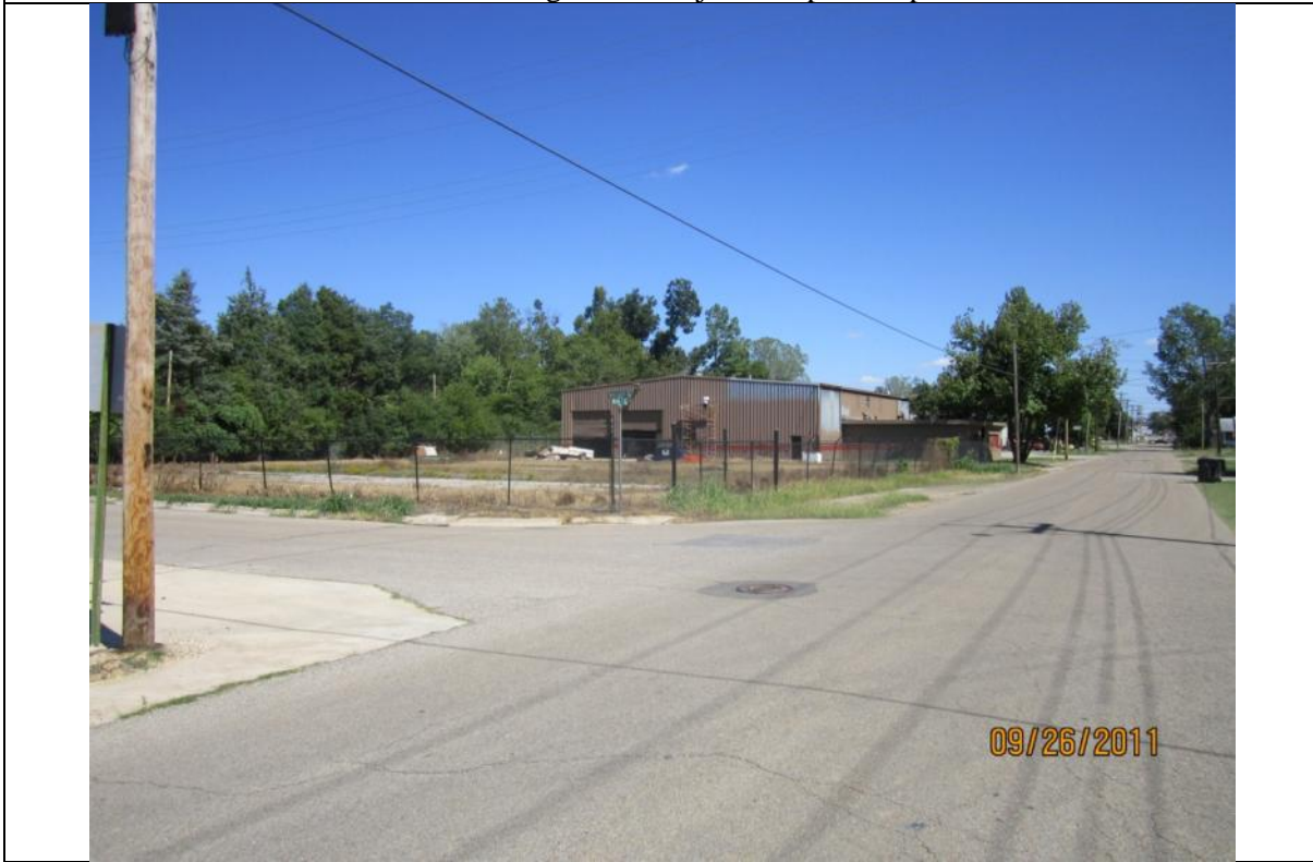
View looking Northeast of subject site parking area and building.
