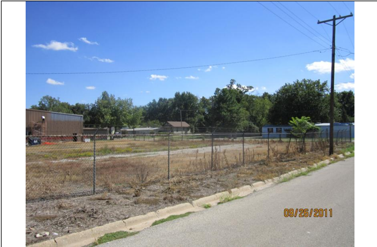
View looking Southeast of subject site parking area and building.
