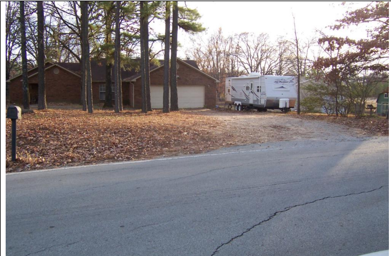
View looking of the subject property along Hudson Dr.
