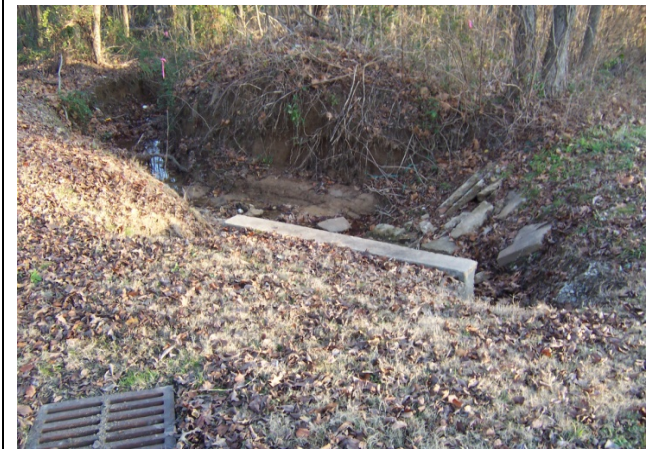
View looking from Harrisburg at Drainage Channel
