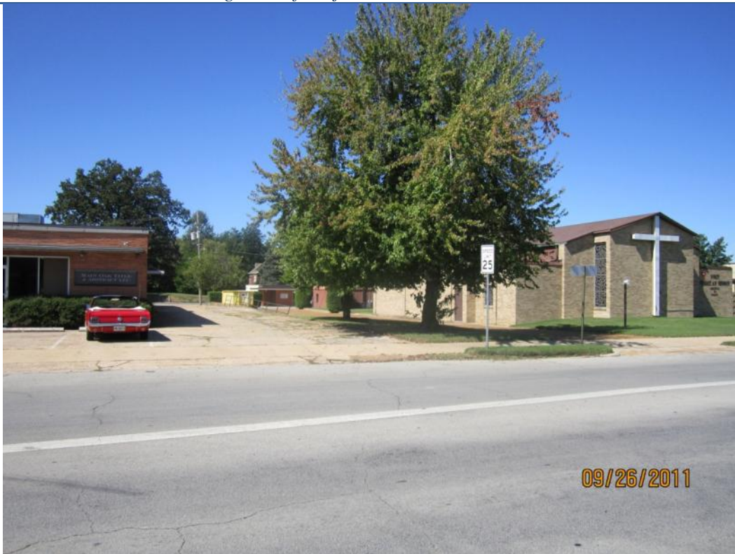
View looking West of abutting Law Office and subject property.
