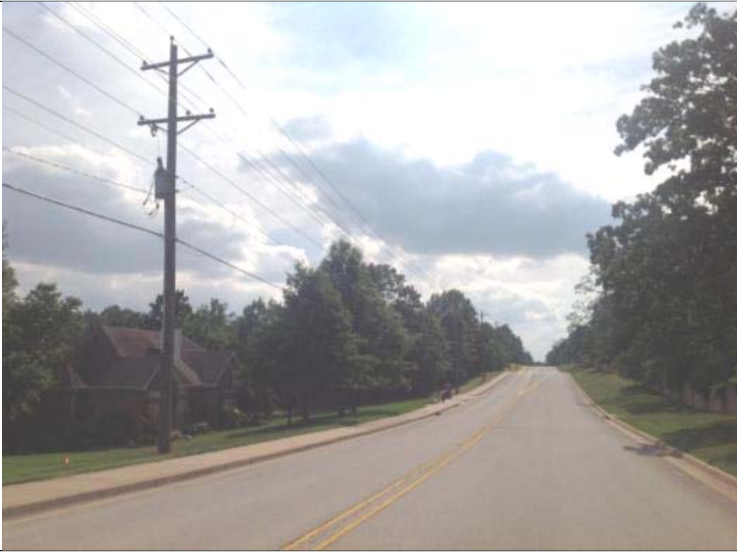
View looking west on Neely Rd.
