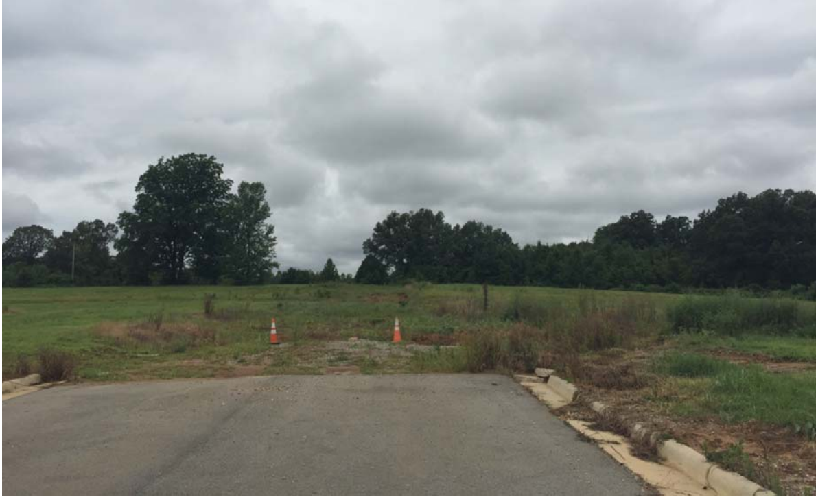
View looking West toward to subject property @ the terminus of Hill Park Dr.
