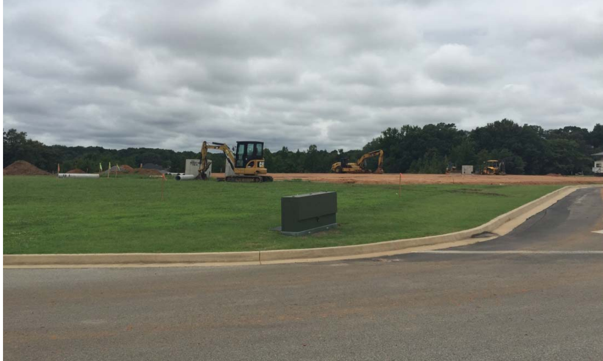
View looking Northwest from Ritter Drive towards the Forest Home Church Campus
