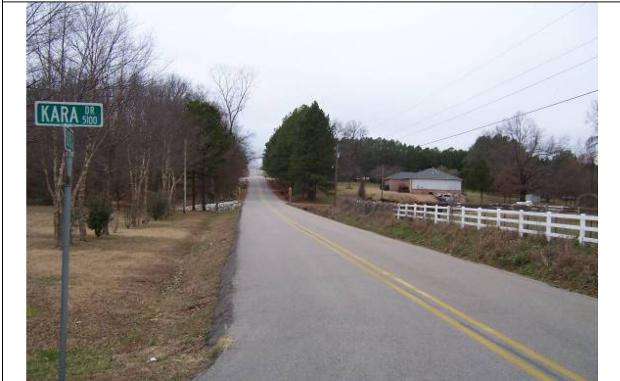
View of the site looking west
