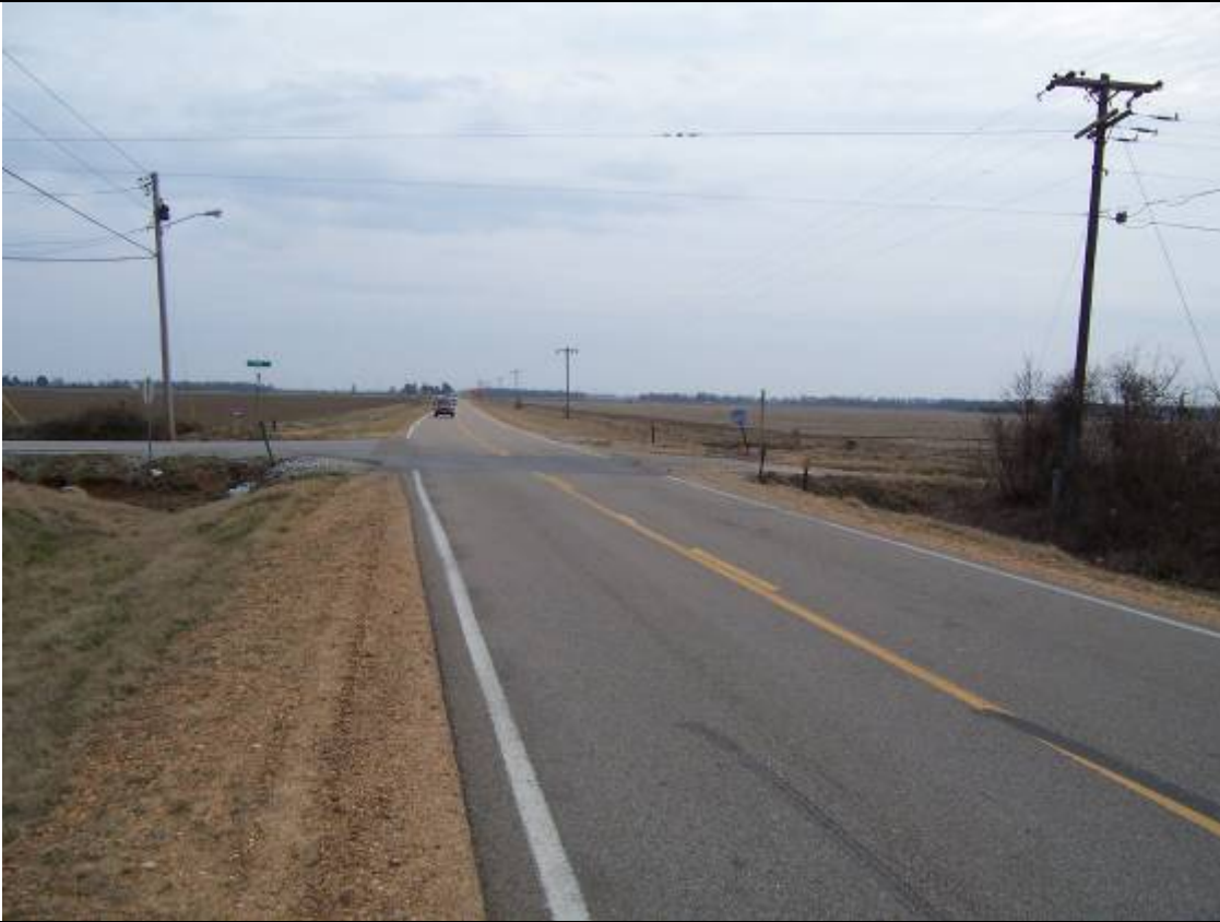
View Looking south along Hwy. 226 @ the intersection of Flemon Rd.
