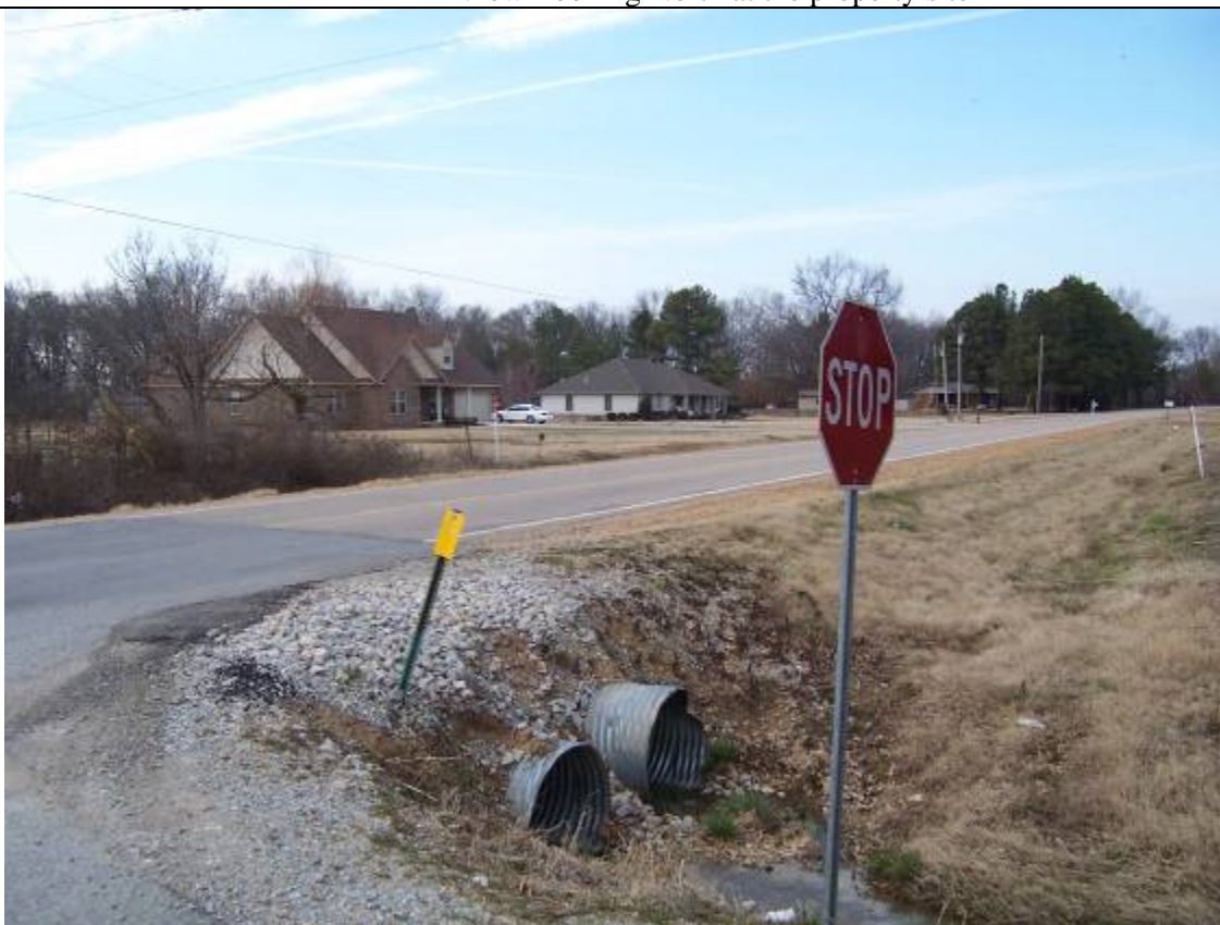
View Looking northwesterly @ the intersection of Flemon Rd. & Hwy. 226
