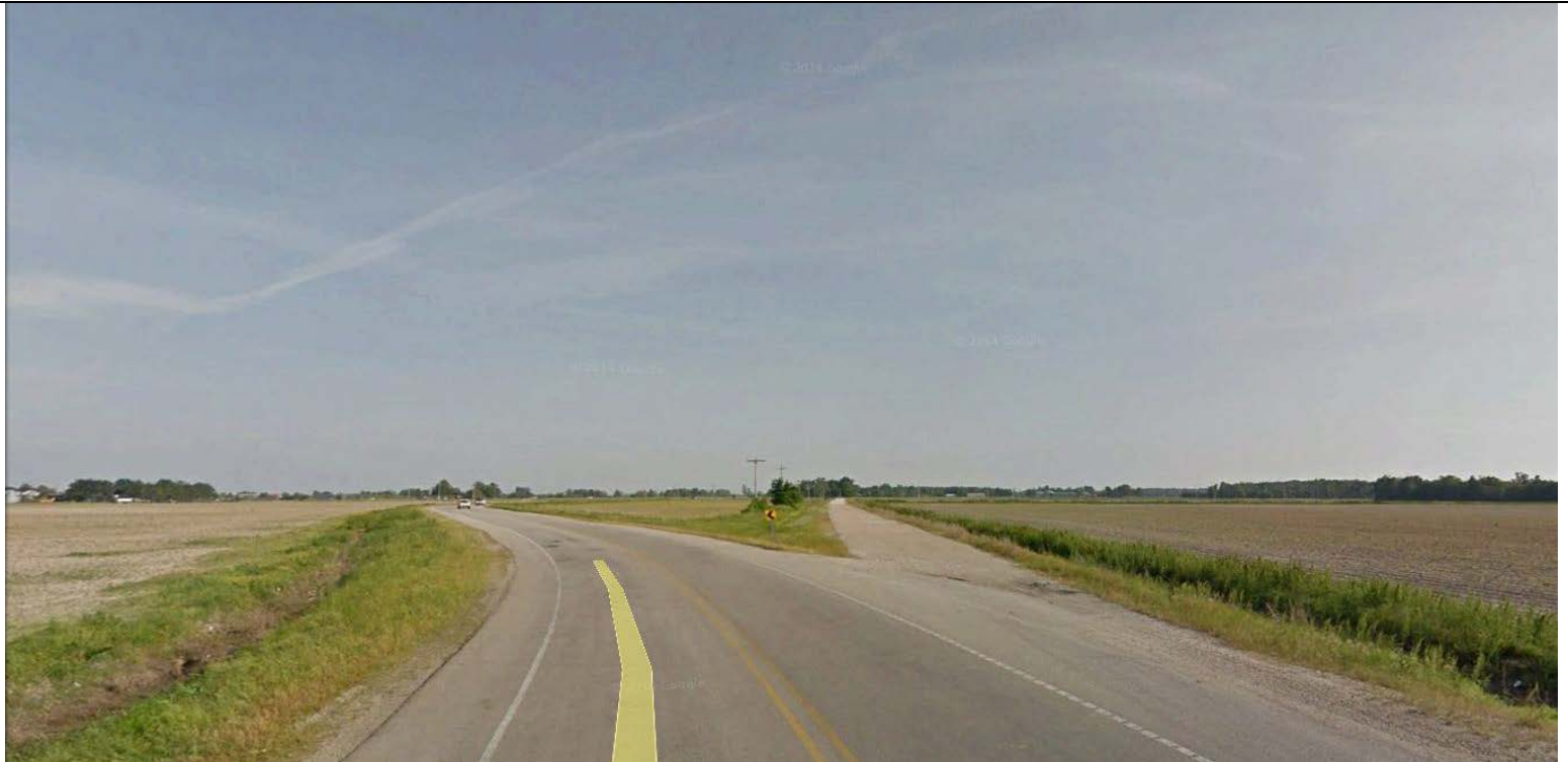
View looking South on Rogers Chapel
