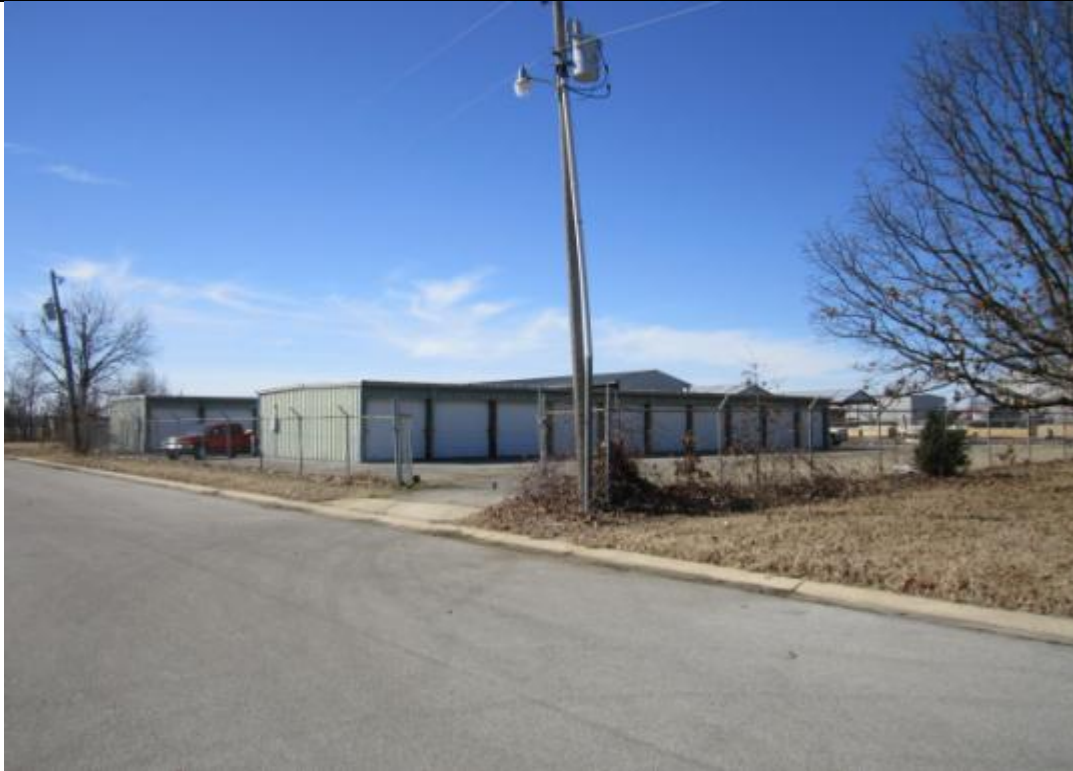
View looking southwest toward subject site.
