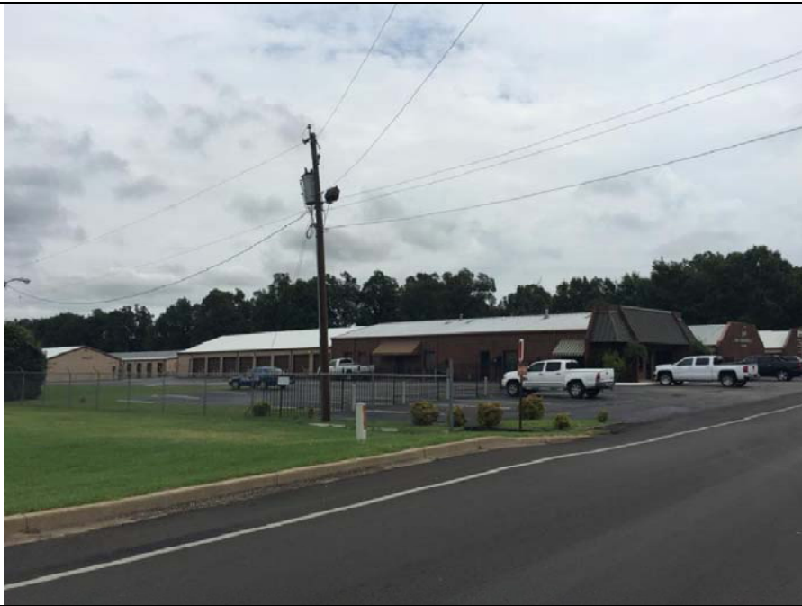
View from Washington looking northeast toward existing Facility
