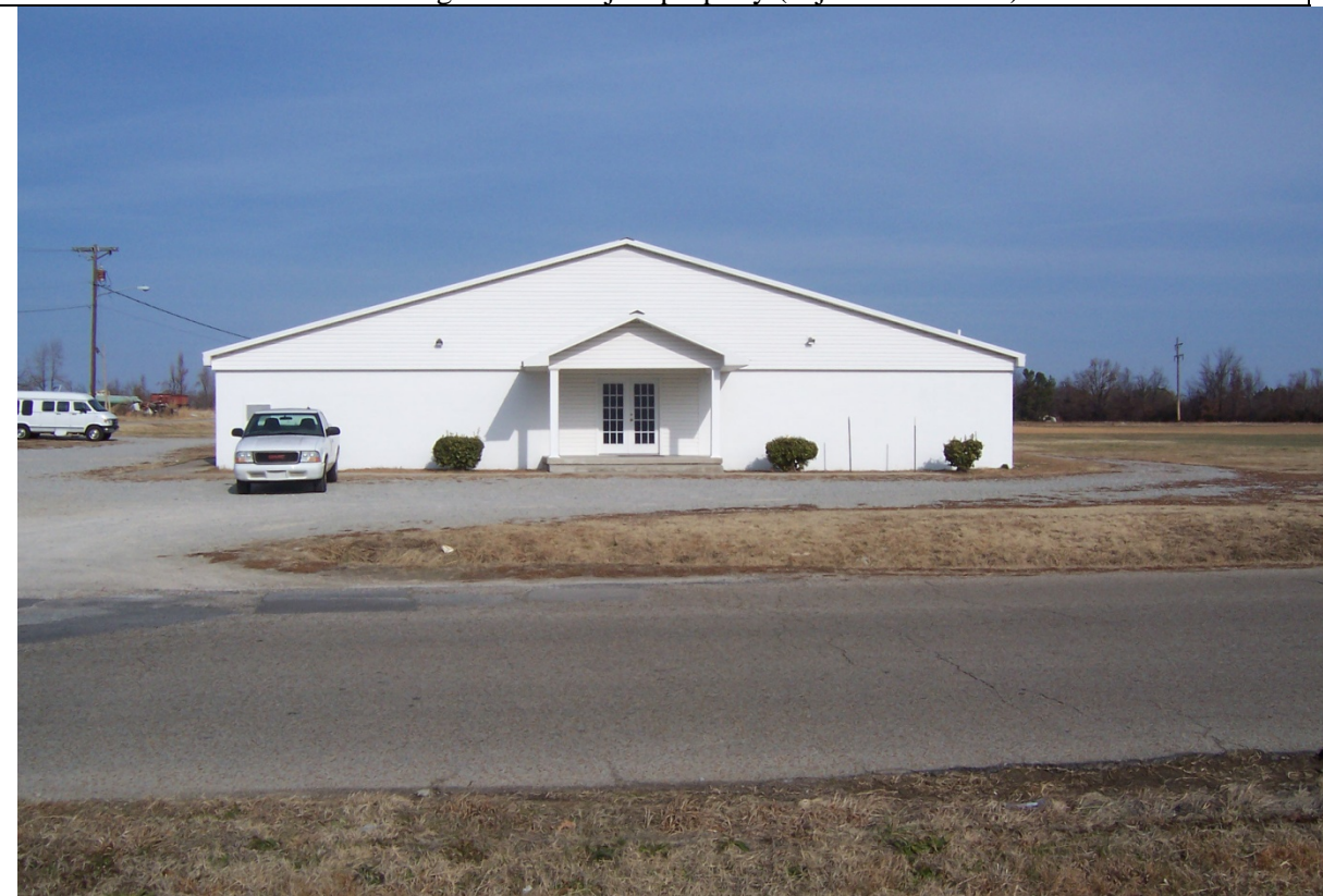
View looking north at church adjacent of subject property (Jonathan Dr.).
