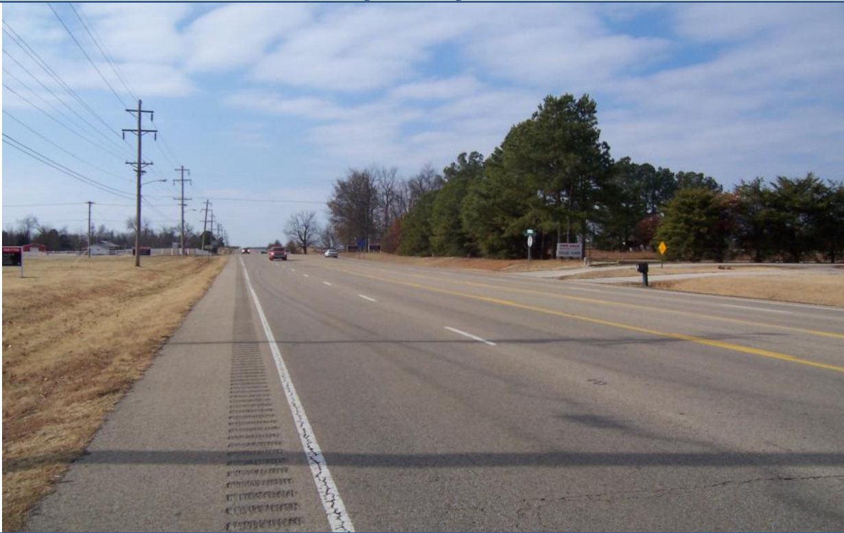
View looking West along Johnson Ave.
