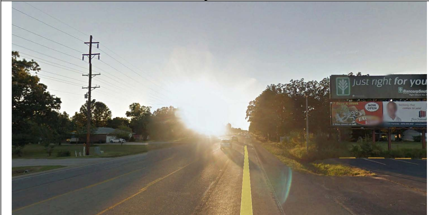
View looking West along E. Johnson Ave.
