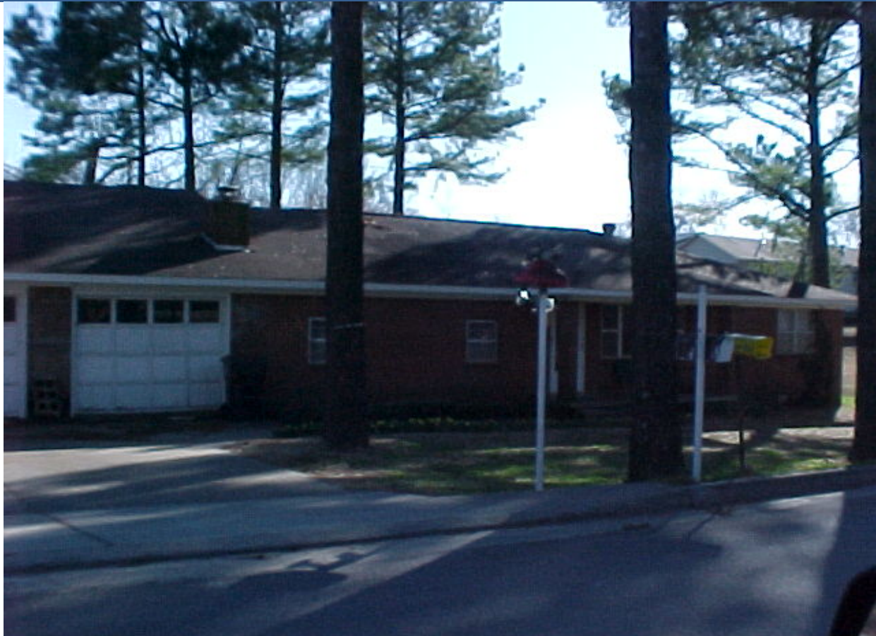
View Looking South at Subject Non-Conforming Structure/Home
