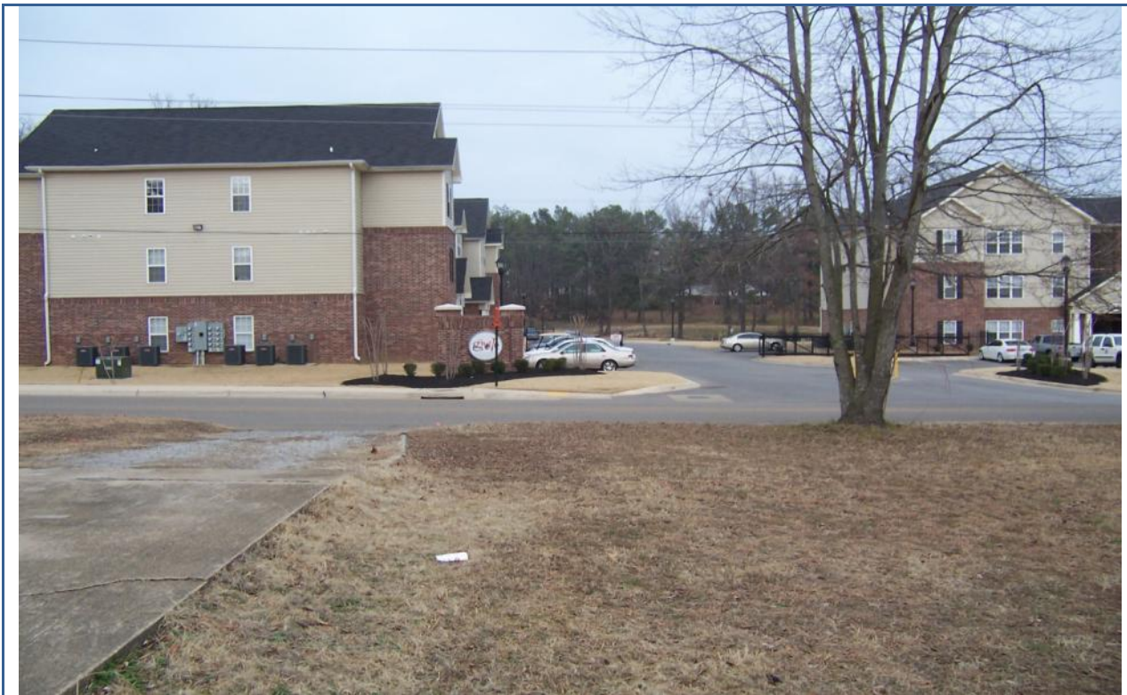
View looking East from rear yard of The Grove Apartments.
