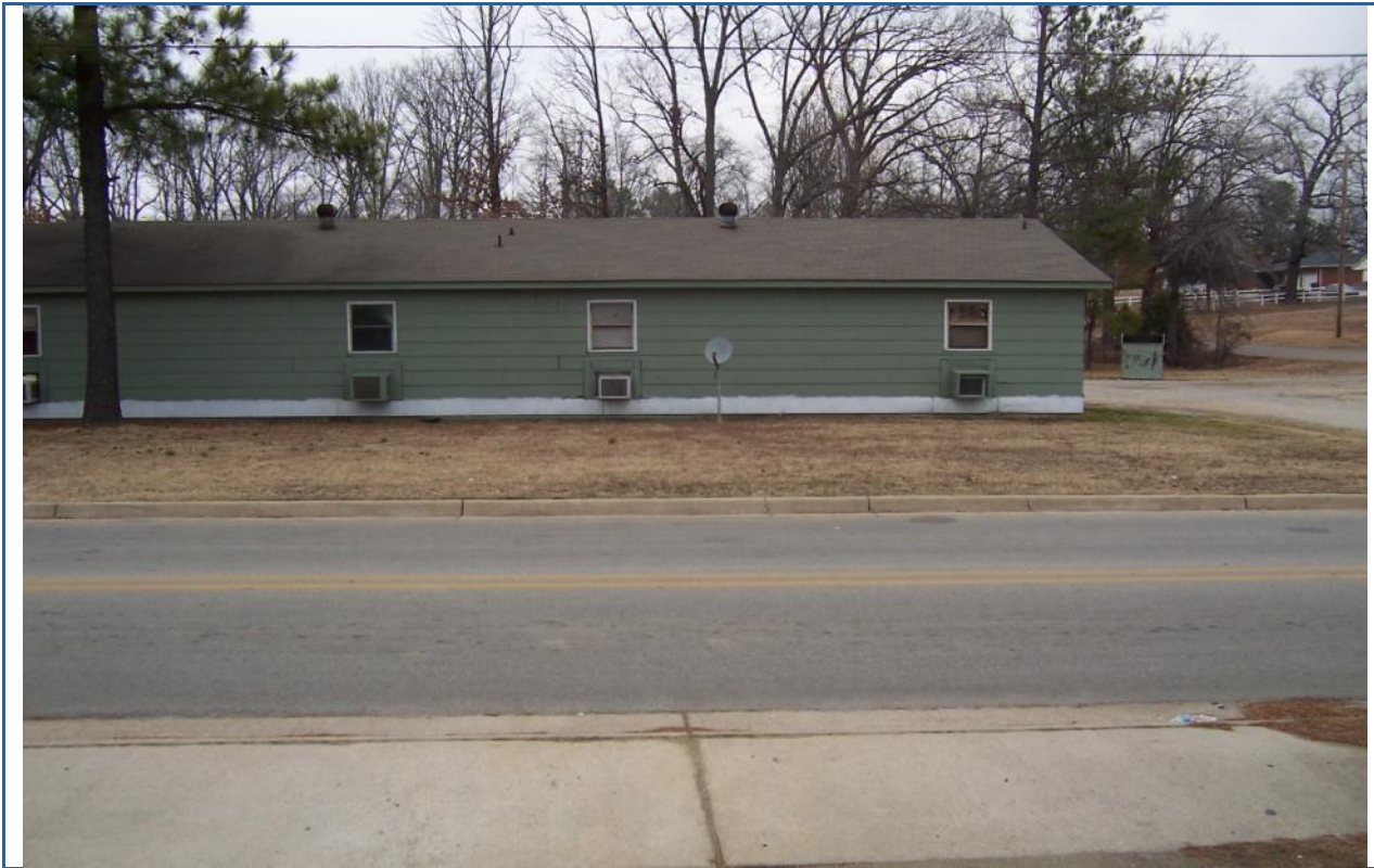
View looking North of adjacent apartments..
