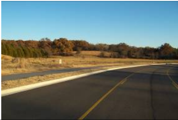
View looking Southeast on Christian Valley Dr. (CVD)
