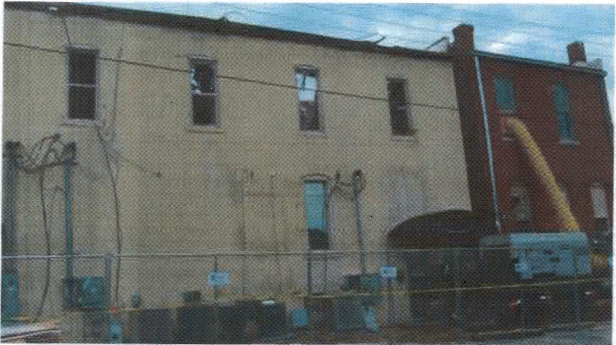
Photo 42 - West face of building.
