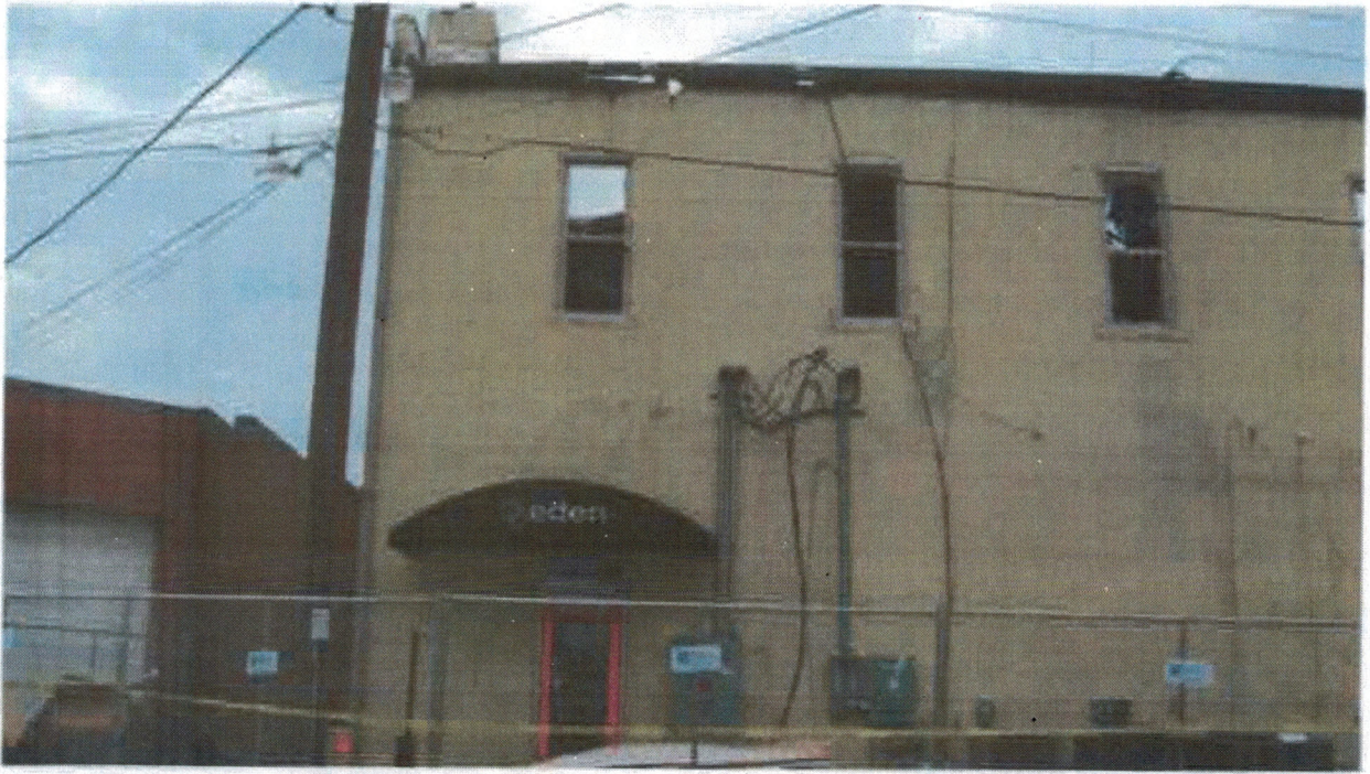
Photo 41 - West face of building.
