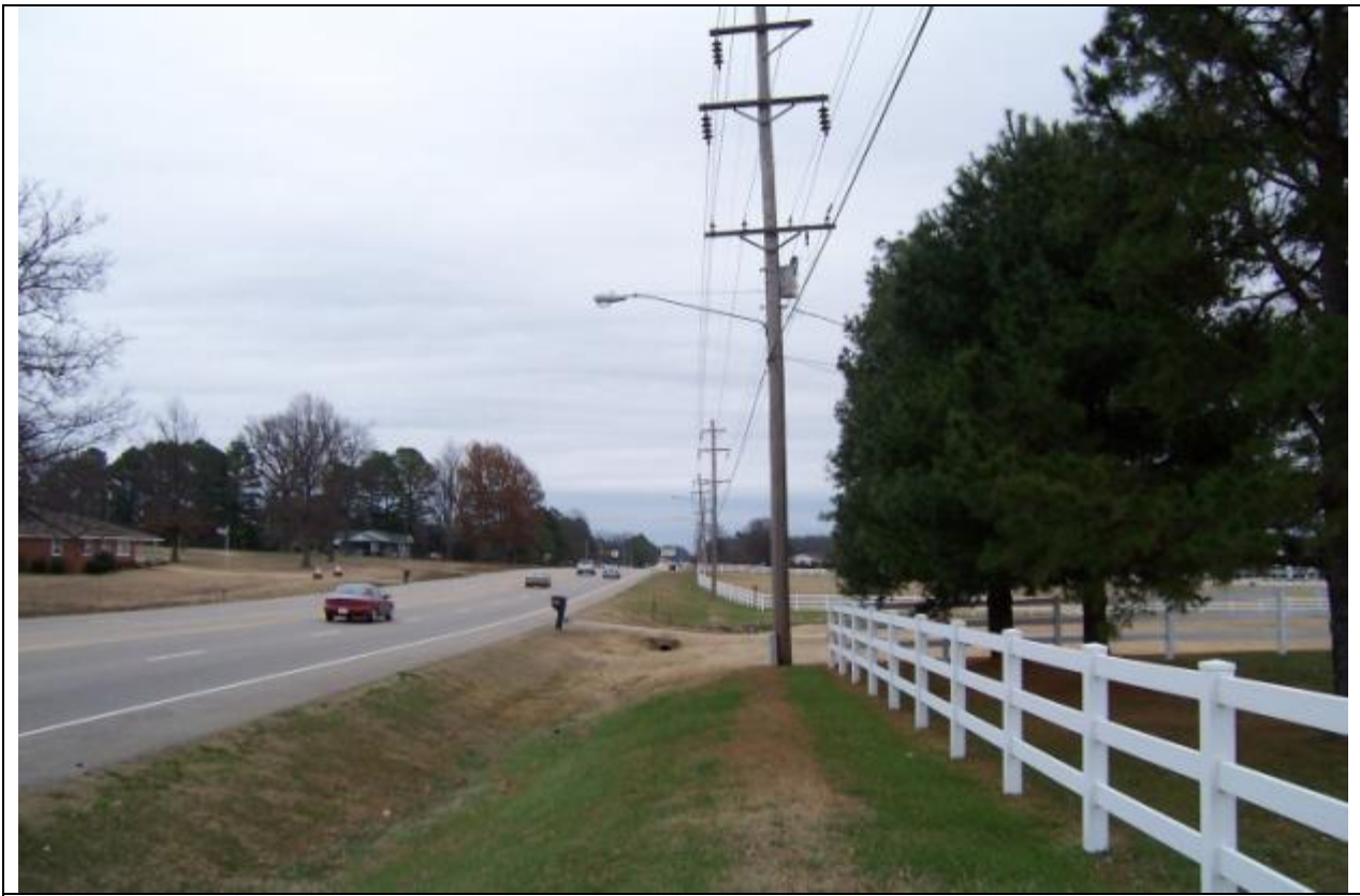
View looking Easterly
