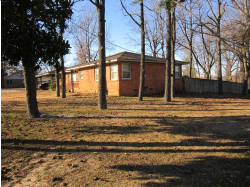
View looking northwest toward 2900 Stalling Lane located west of site.
