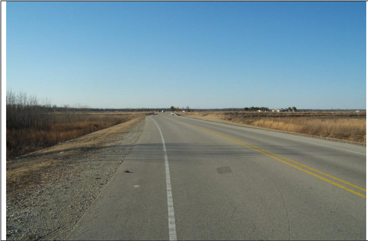
View looking north along frontage (Nestle Road).
