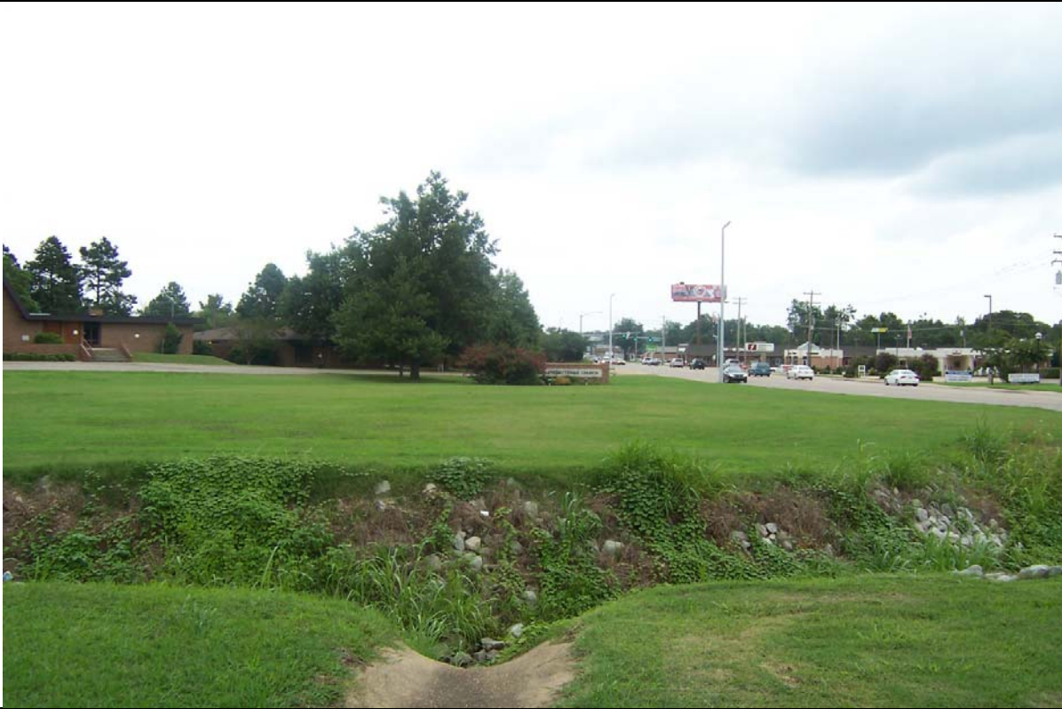
View Looking Northeast from site
