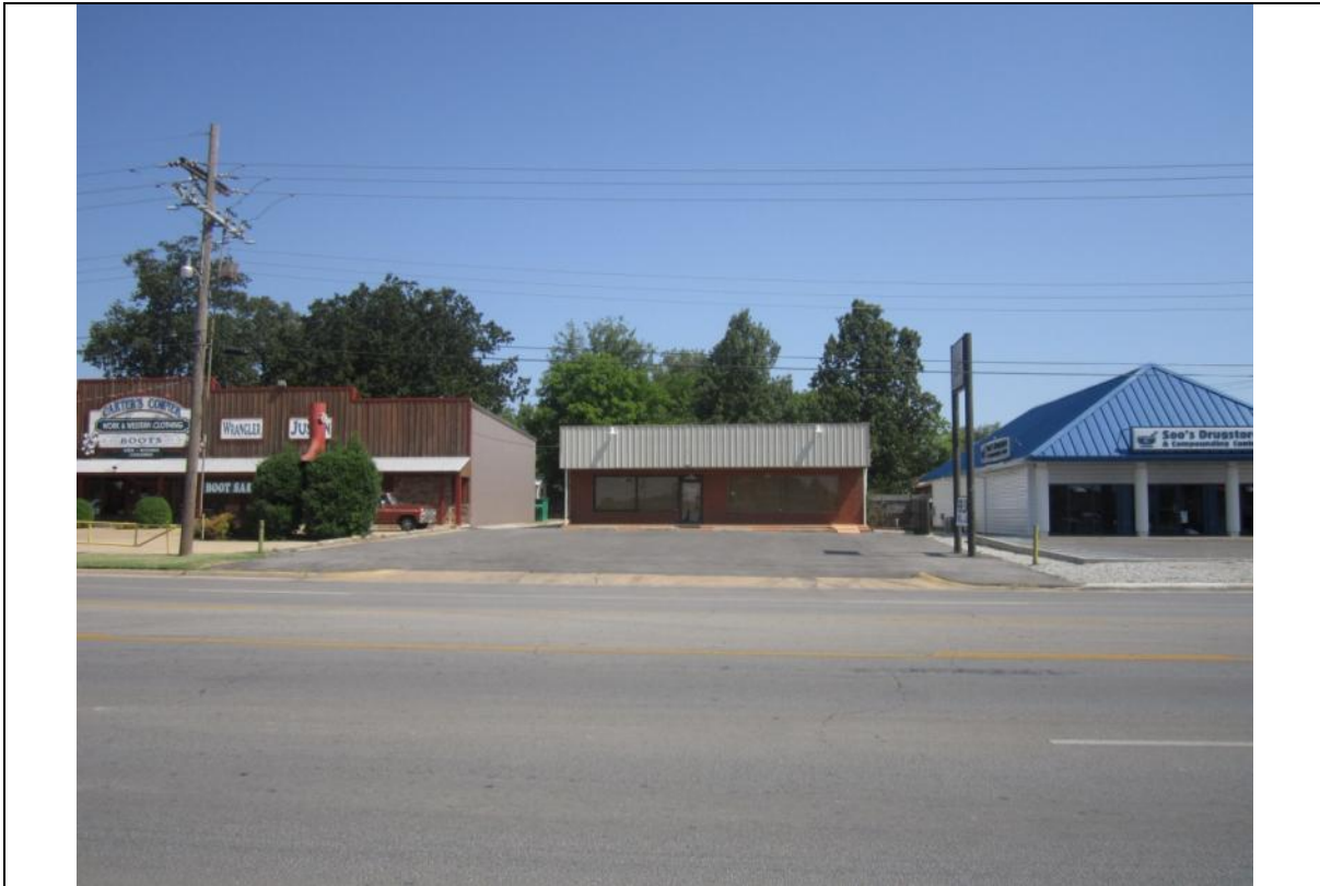
View looking North at the subject property along E. Nettleton Ave.
