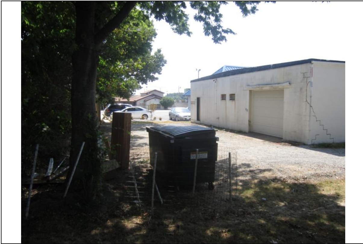
View looking East from rear property line.
