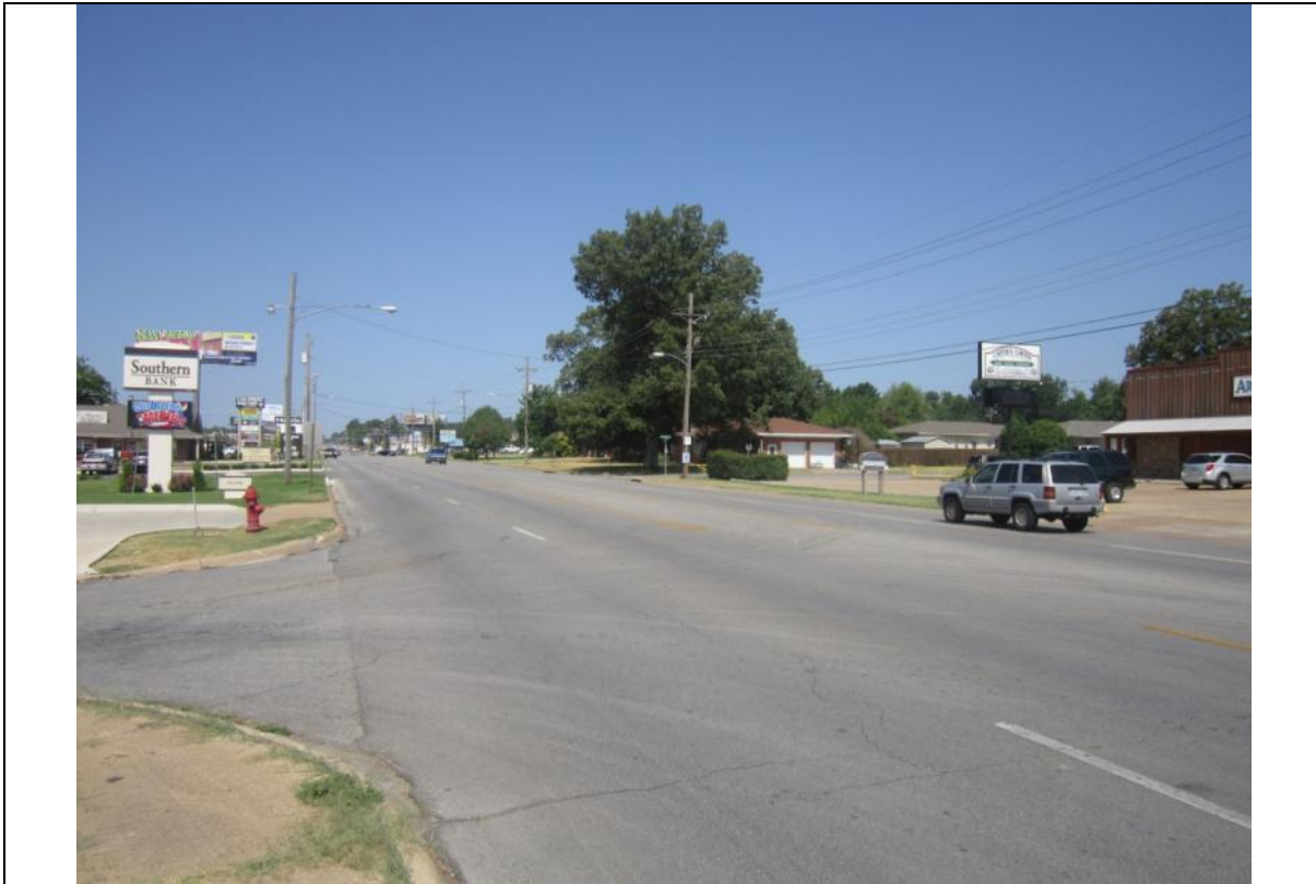
View looking West along E. Nettleton Ave.
