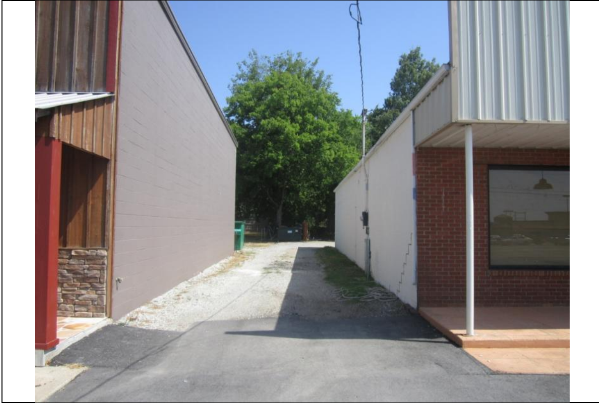
View looking North along west wall of subject property.
