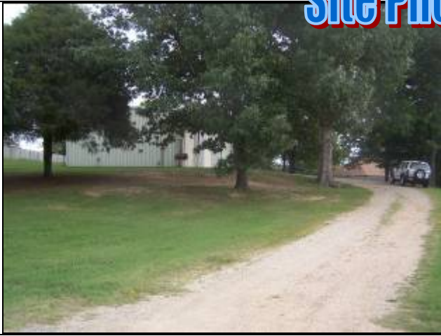
View looking East at subject building
