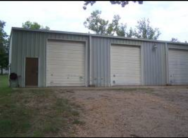
View looking North at subject building
