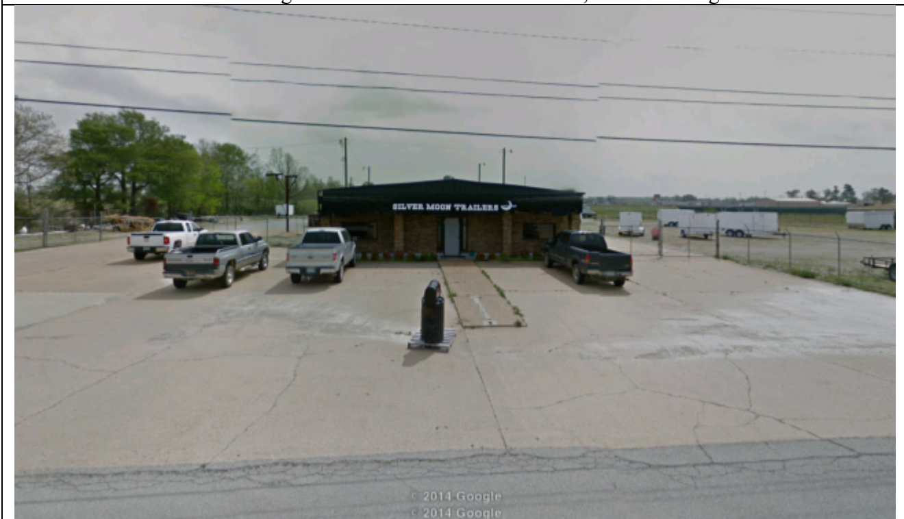
View looking east toward subject property
