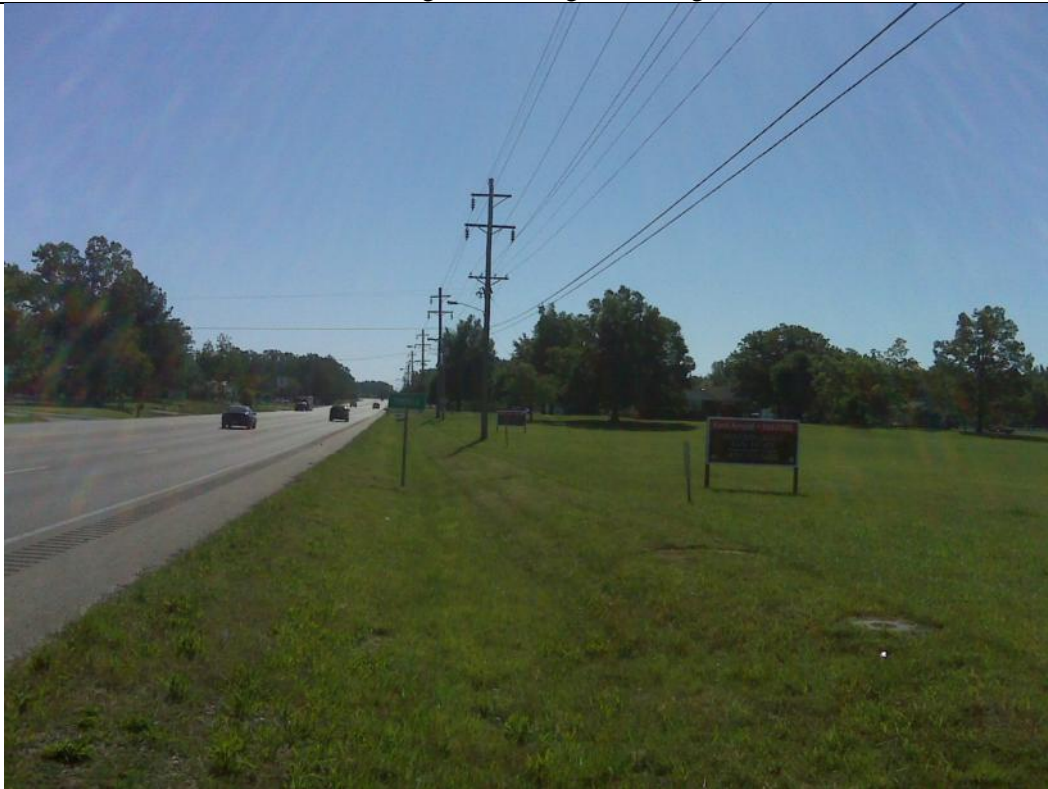
View looking to the east along Hwy. 49 N Frontage
