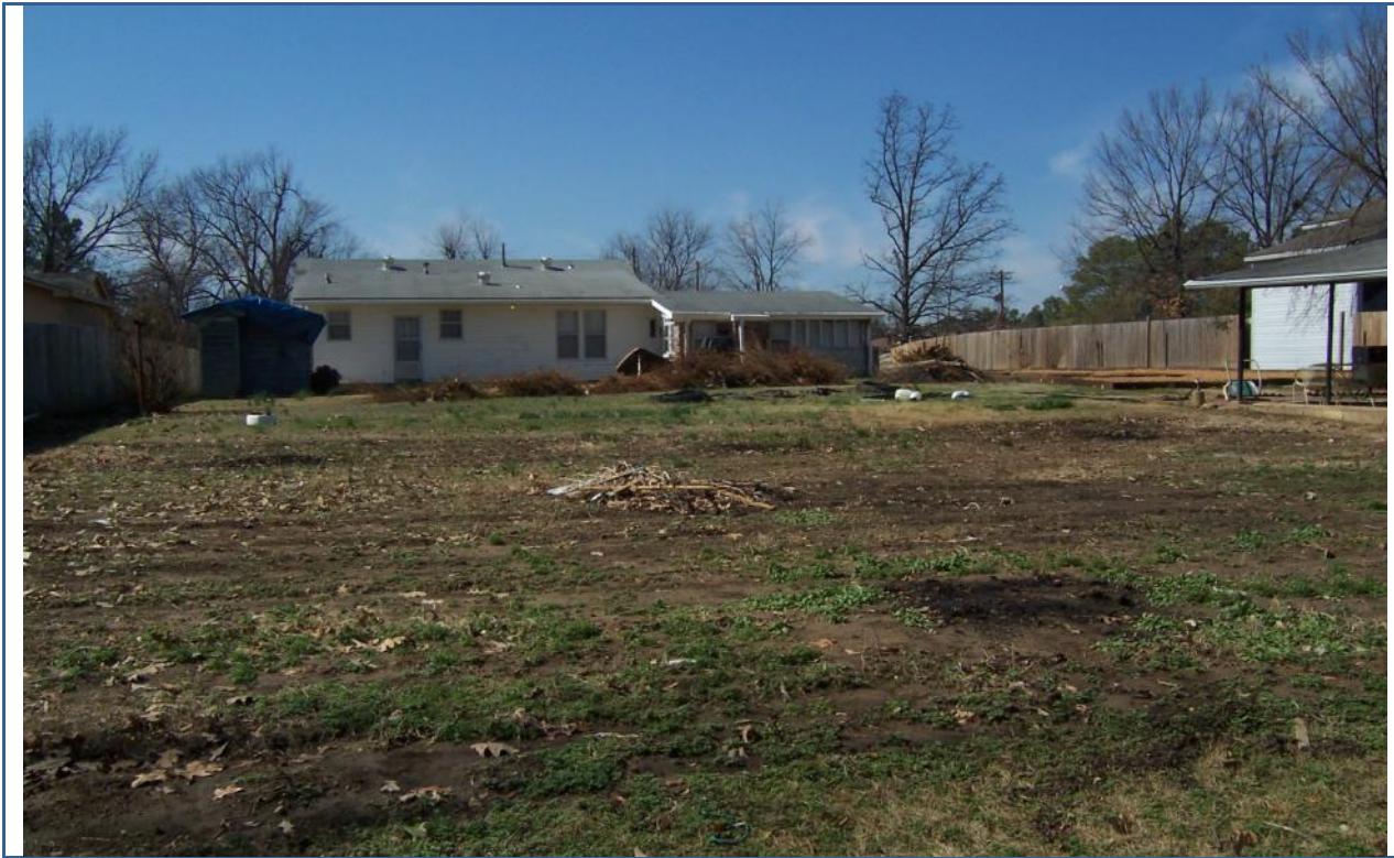
View Looking West at Subject Structure/Home (rear).
