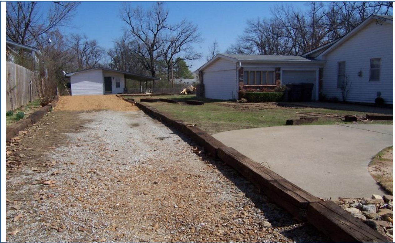
View looking East of secondary structure and driveway.
