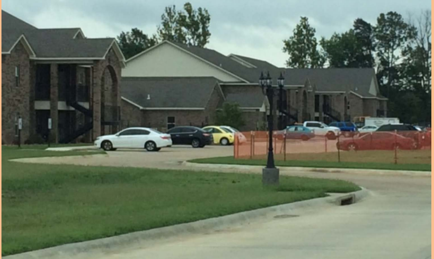
View looking Southeast toward apartments
