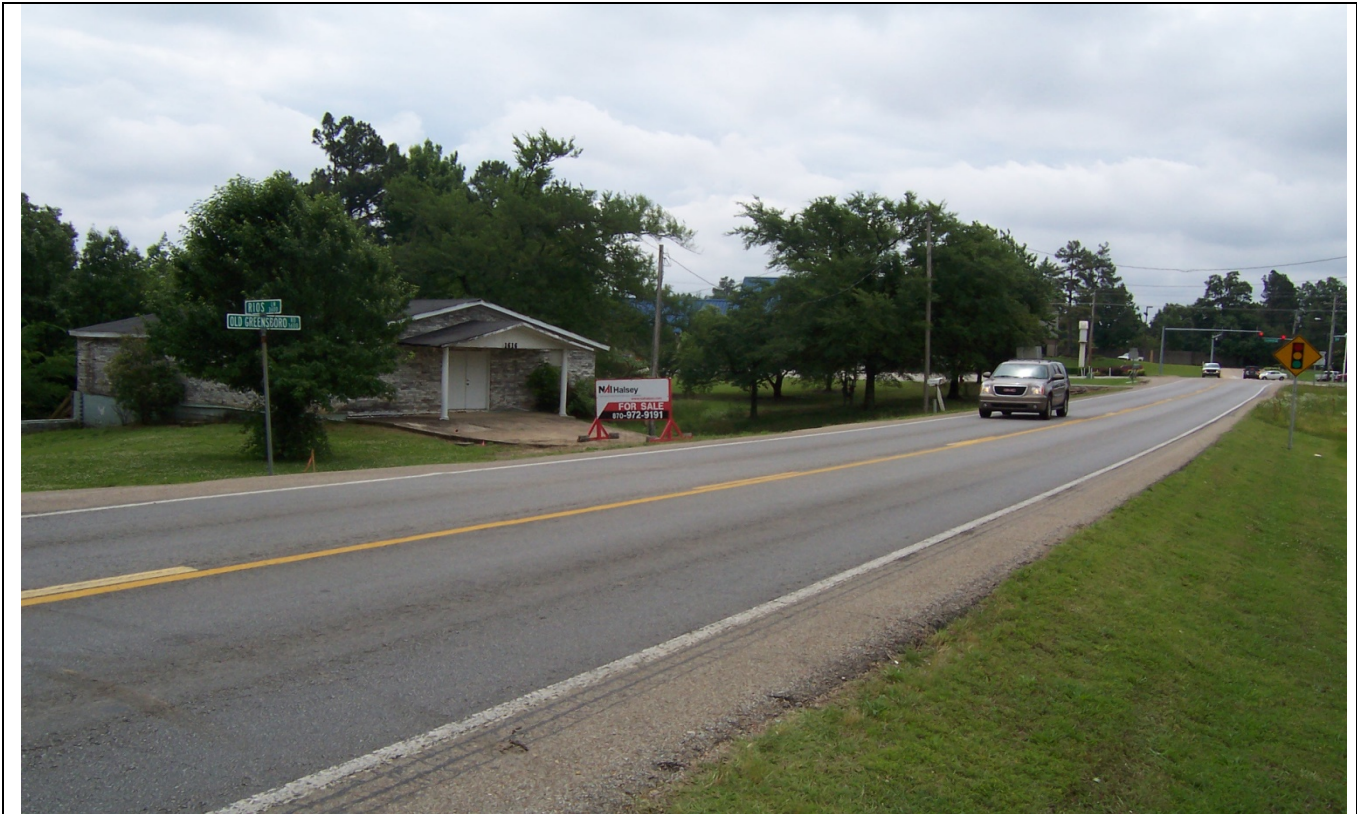
View looking to the east along Old Greensboro Rd of C-3 L.U.O. property.
