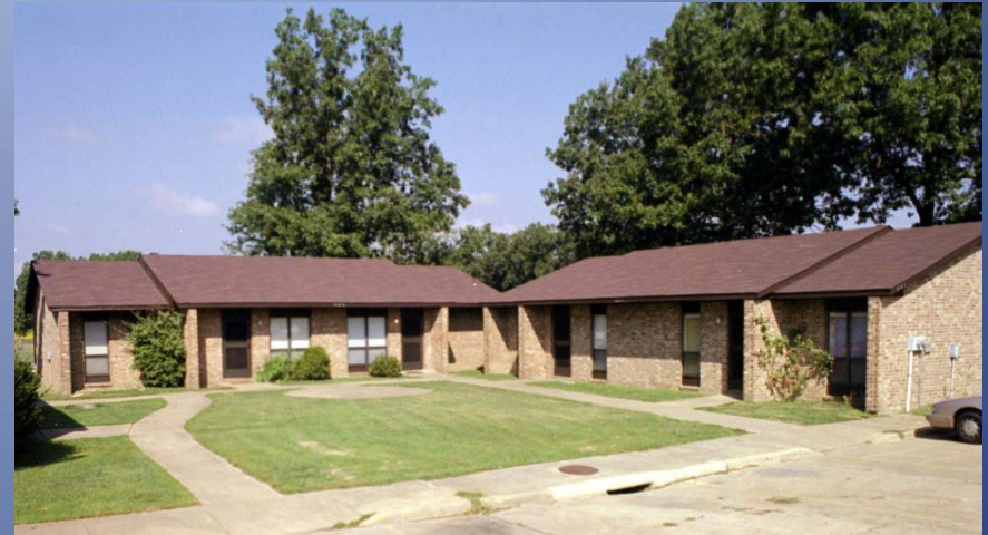
Cayman Villa-46 Family Units Located on Alpine Street
