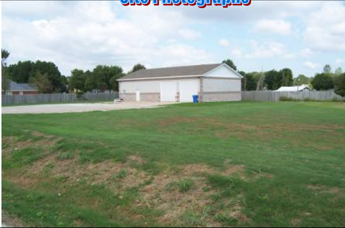
View looking Northeast at subject building
