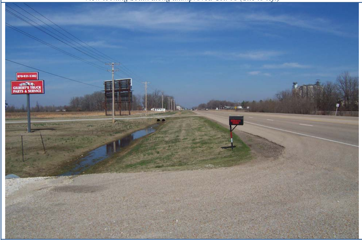
View looking Northeast along Hwy 49N
