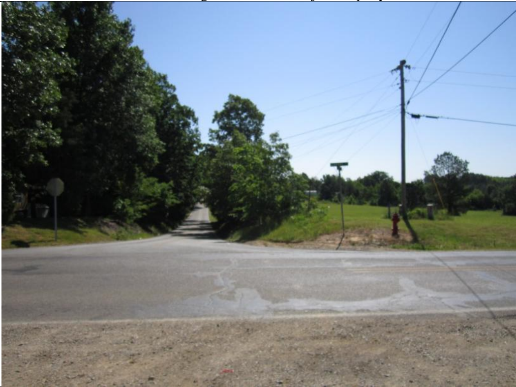
View looking East towards Prospect Rd./ Subject Property to Right
