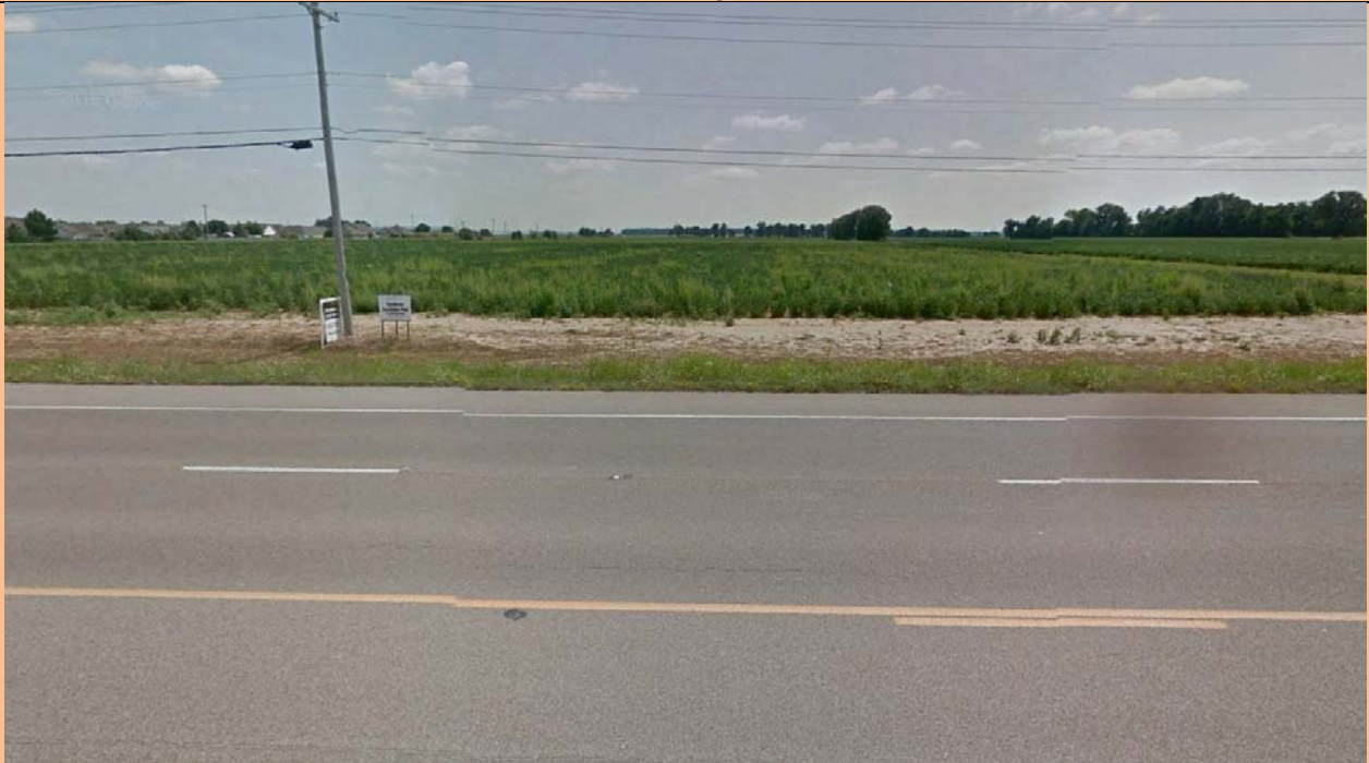
View looking South
