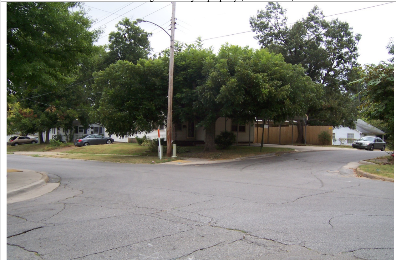
View looking southeast of subject property.
