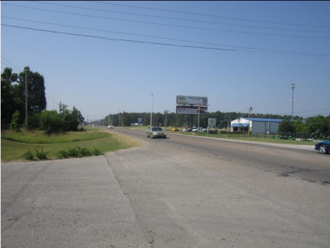
View of looking South along Stadium Blvd.
