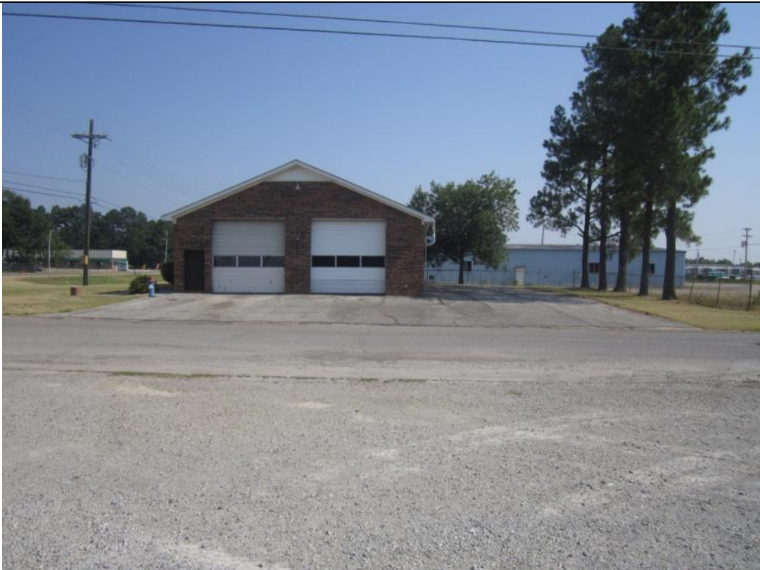
View looking North from adjacent property.
